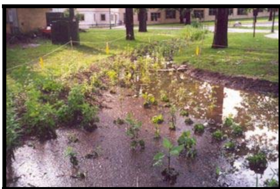
Newly Constructed Bioretention Area
