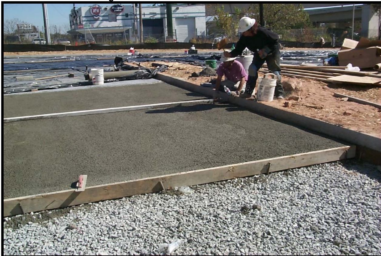
Figure 4-54. Porous Pavement Installation
