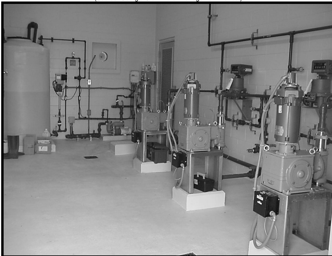
Figure 4-66. Dosing/Injection Components of an Alum Treatment System
