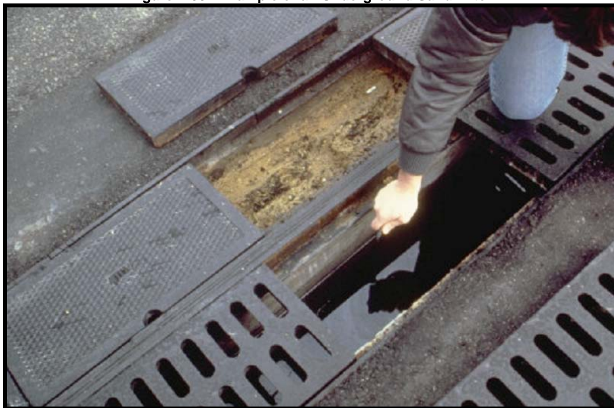
Figure 4-59. Example of an Underground Sand Filter
