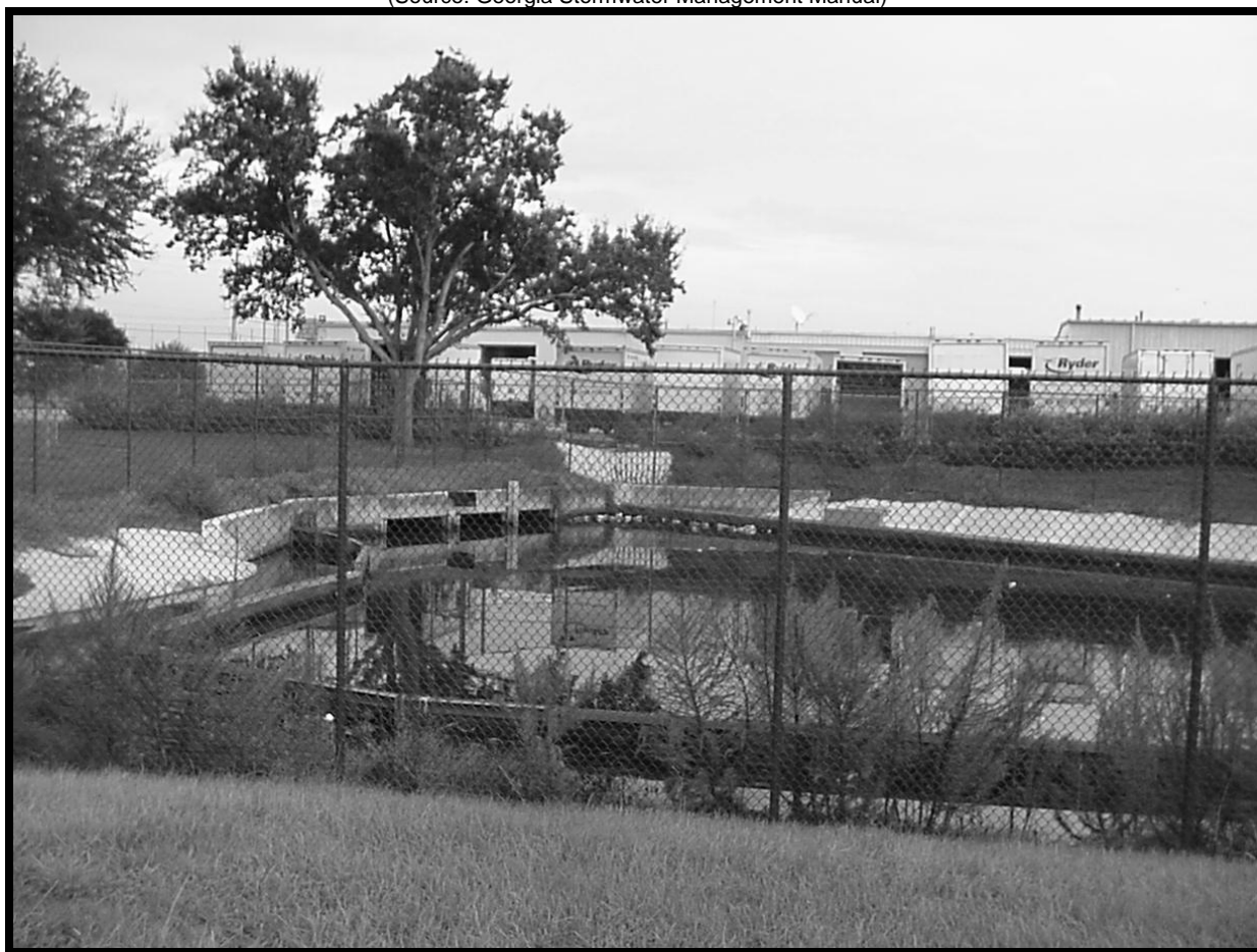
Figure 4-65. Settling Basin for an Alum Treatment System
