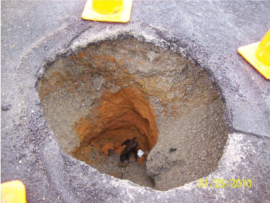
Drainpipe failure on Freshour Street.
