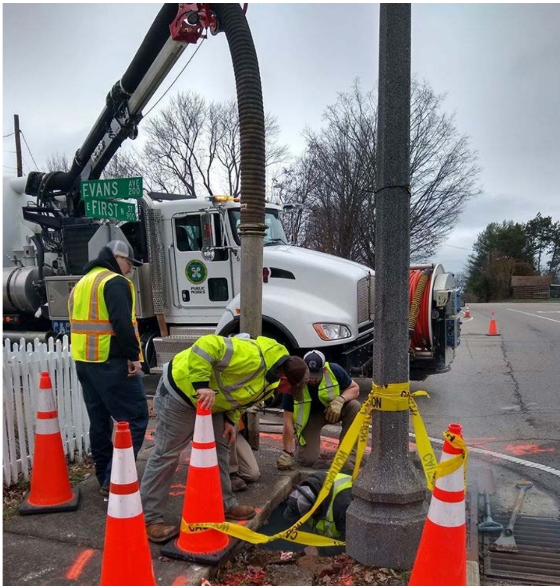
Crews making repairs to storm water system
