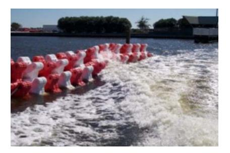
Figure 3-8 Floating wave attenuation device<sup>17</sup>
