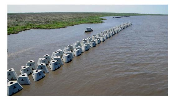
Figure 3-7 Wave attenuation devices<sup>16</sup>
