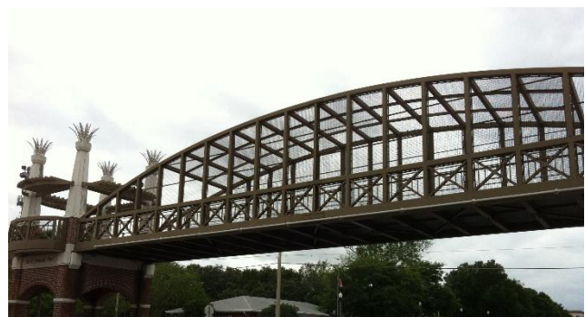
West Orange Trail Bridge (source: DRPMO)
