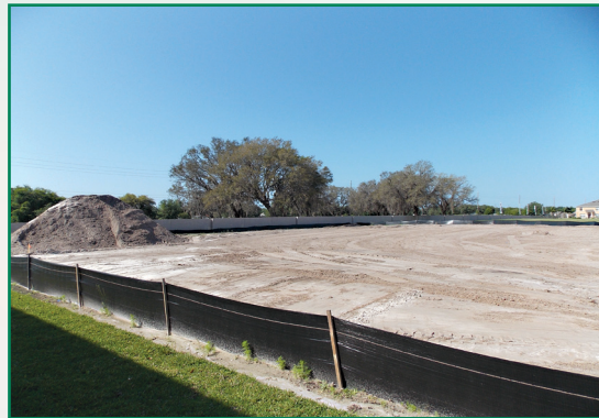
Silt Fence at Construction Site
