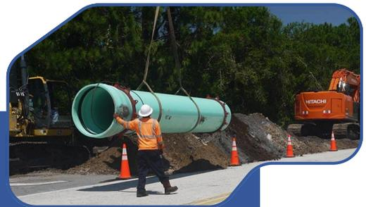
Figure 34. A Stormwater Pipe Ready to be Installed in Tampa, Florida (Source: City of Tampa).
