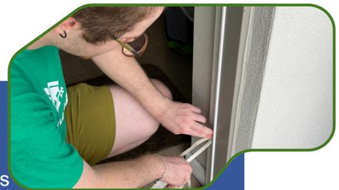
Figure 53. Weatherstripping Being Performed by EnergyUpgrade (Source: Sarasota County).
