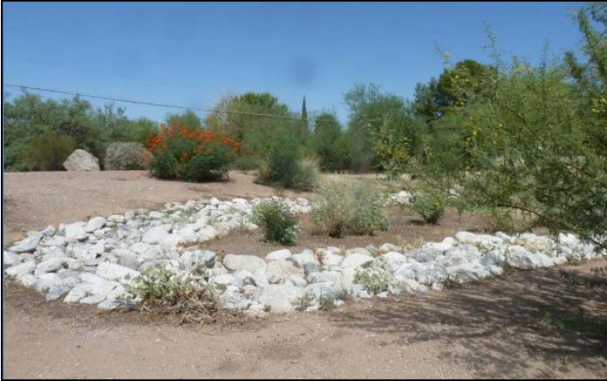
Figure 2-21. Infiltration Trench
