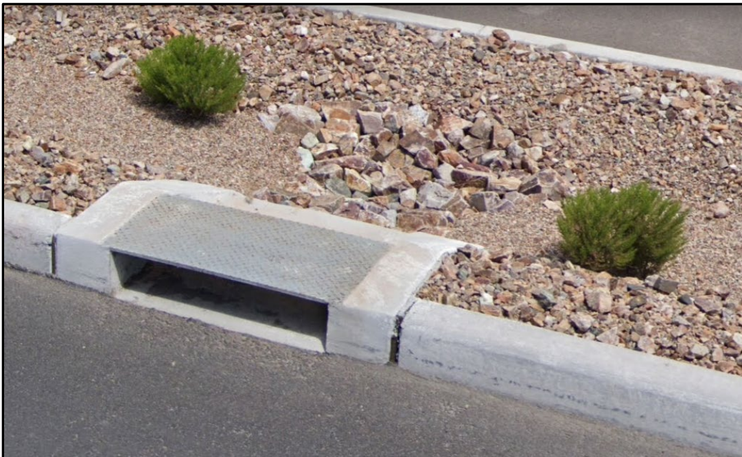
Figure 2-10. Curb opening Type 1, Grant Rd., Tucson, AZ
