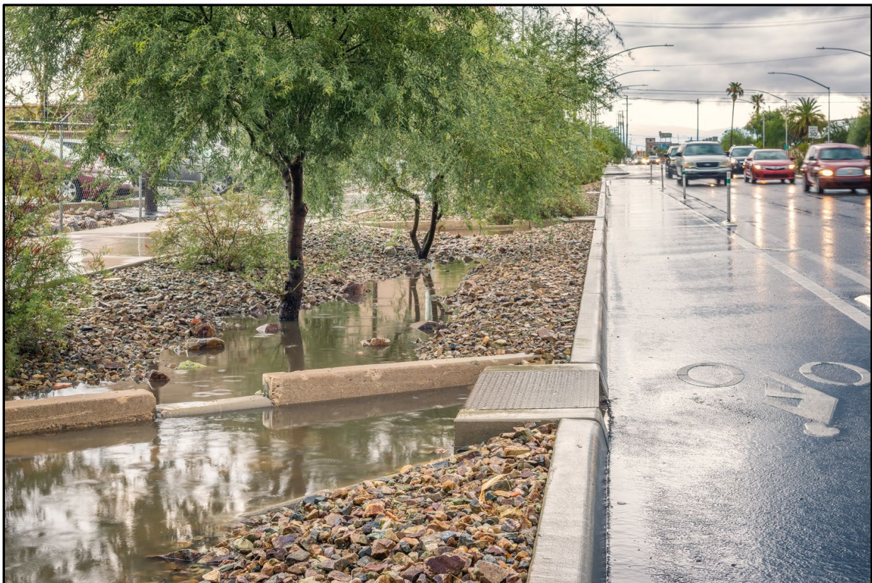
Figure 2-28. Saint Mary's Road Concrete Check Dam
