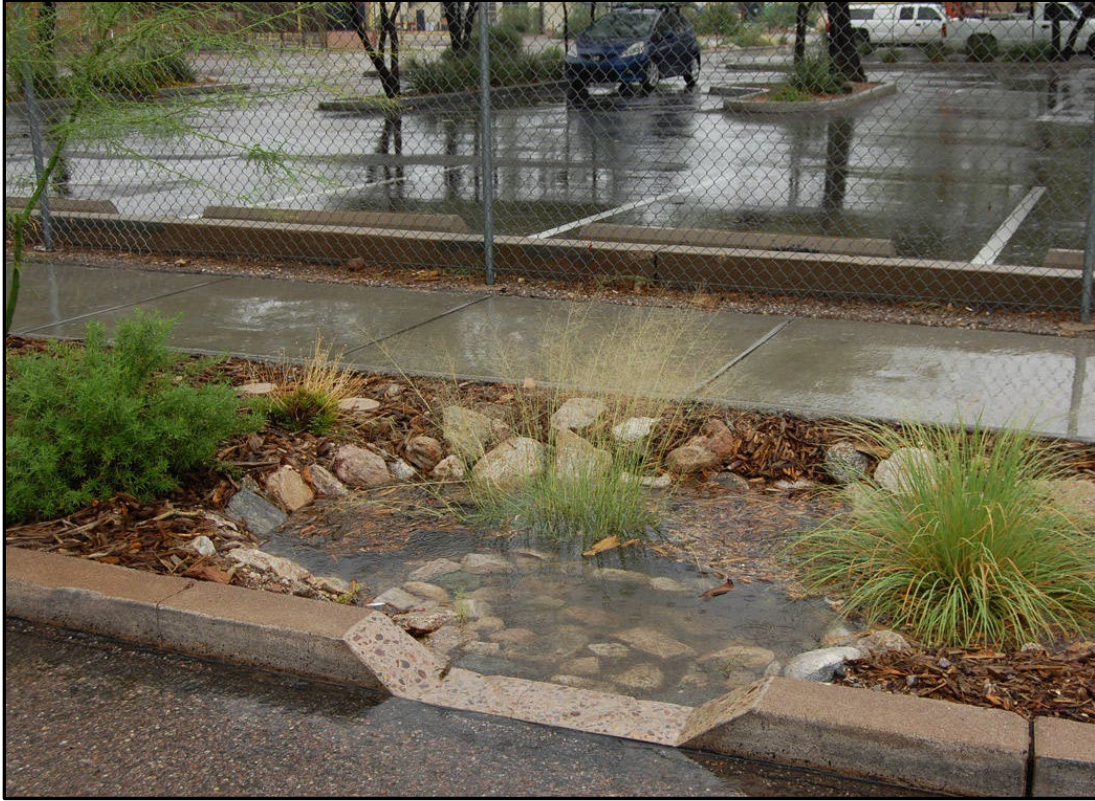
Figure 2-12. Type 2 Curb Retrofit, Tucson Association of Realtors
