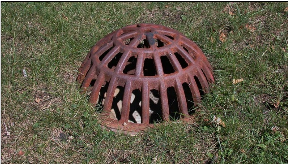
Figure 2-23. Dome Overflow Grate Flush With the Surface
