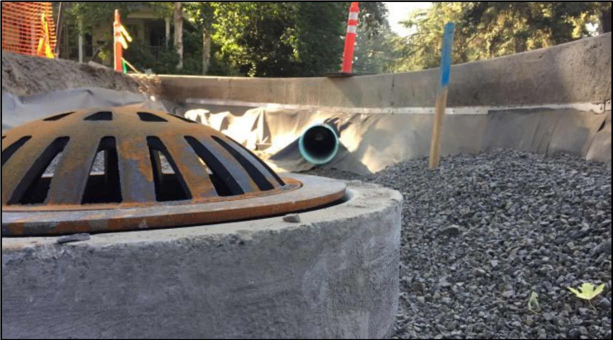
Figure 2-24. Dome Overflow With Riser
