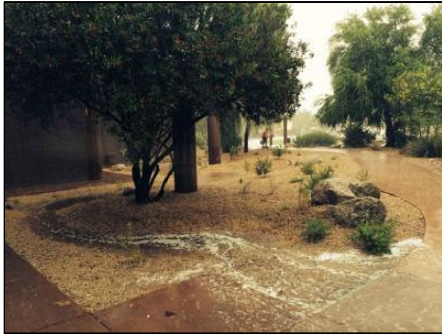
Figure 2-26. Vegetated Swale Near Glendale Arizona Public Library Entrance
