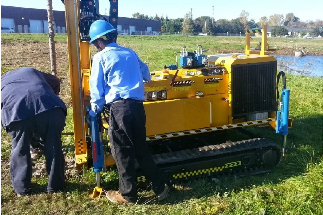
Figure 2-57. Installation of Parjana's IRIS to Promote Infiltration in an Athletic Field
