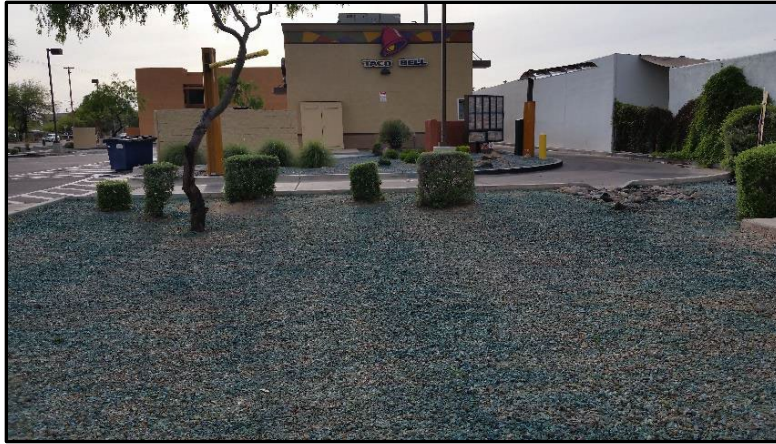
Figure 3-2. A Commercial GSI Installation Sprayed for Weeds and Excessively Pruned
