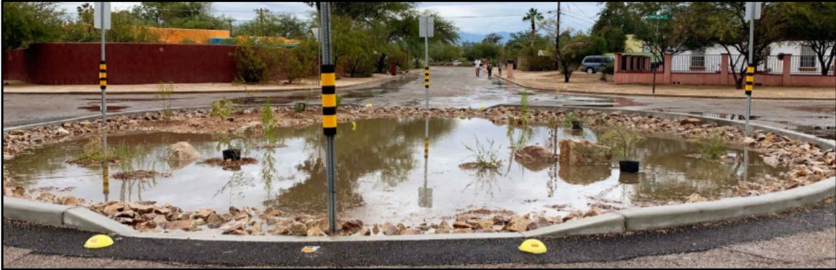
Figure 2-42. Newly Planted Traffic Circle
