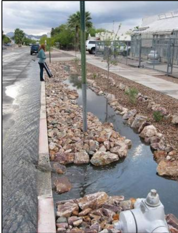
Figure 2-3. Rocked Streetside Stormwater Harvesting Basin
