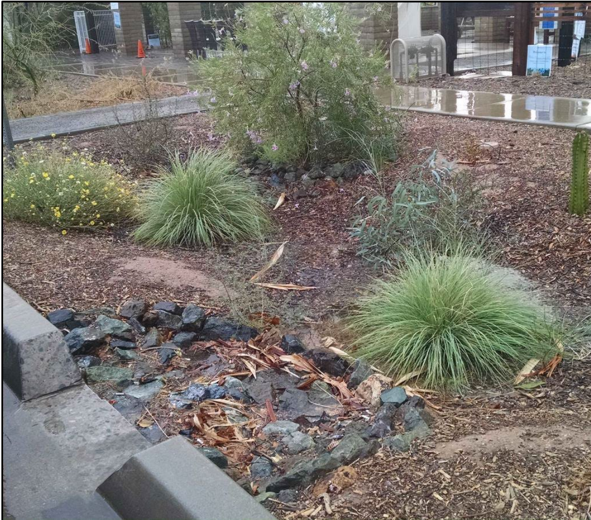
Figure 2-7. Mesa Urban Garden Rock Sediment Trap
