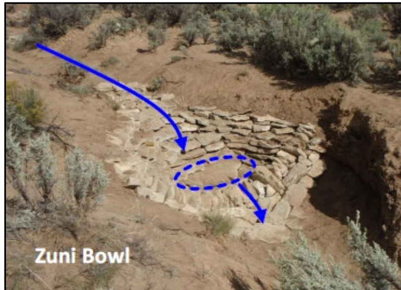
Figure 2-34. Photo of Zuni Bowl Showing the Flow Path
