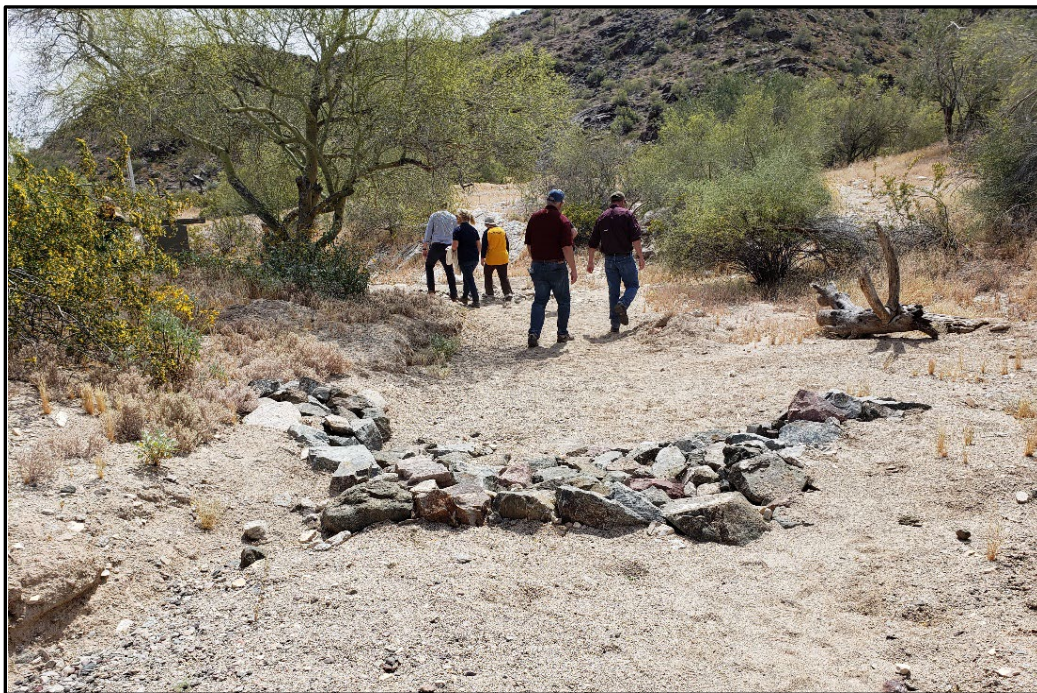
Figure 2-30. One Rock Dam
