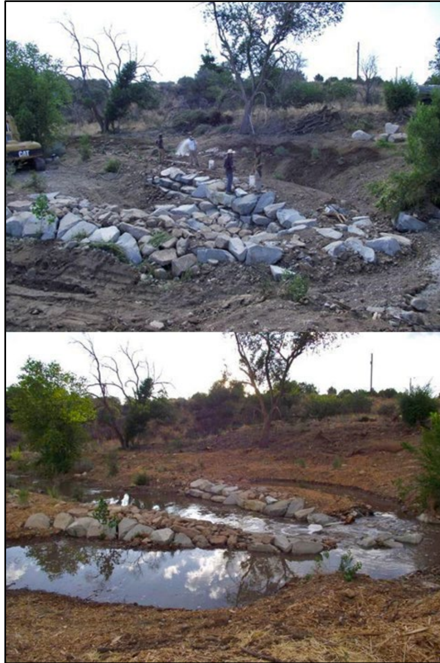
Figure 2-35. During- and Post-Construction of a Large Zuni Bowl
