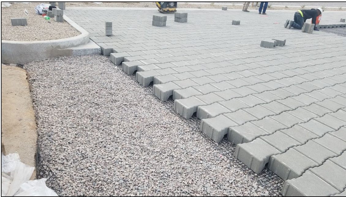
Figure 2-53. Example Permeable Block Installation
