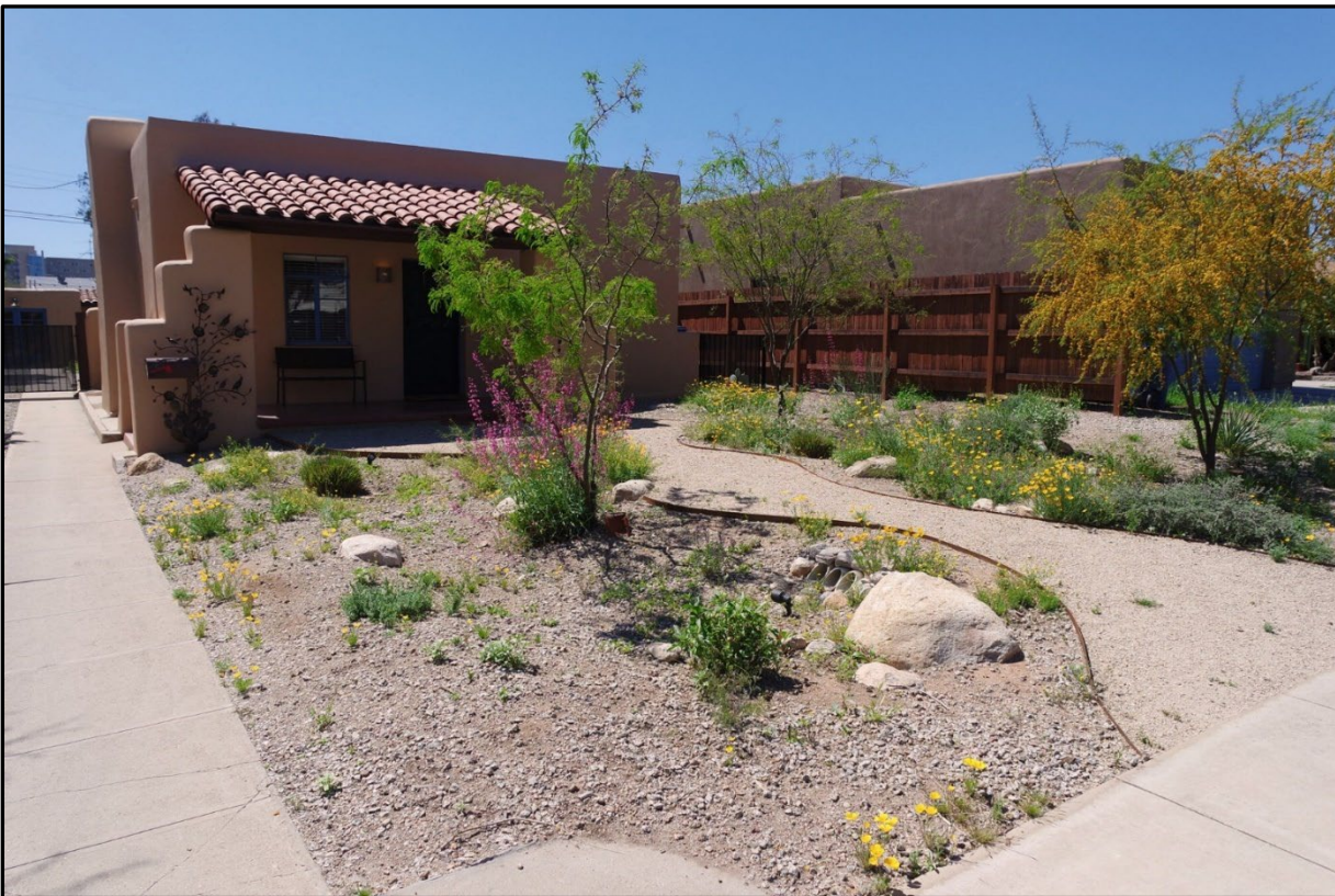
Figure 2-19. Shallow Residential Bioretention Basin
