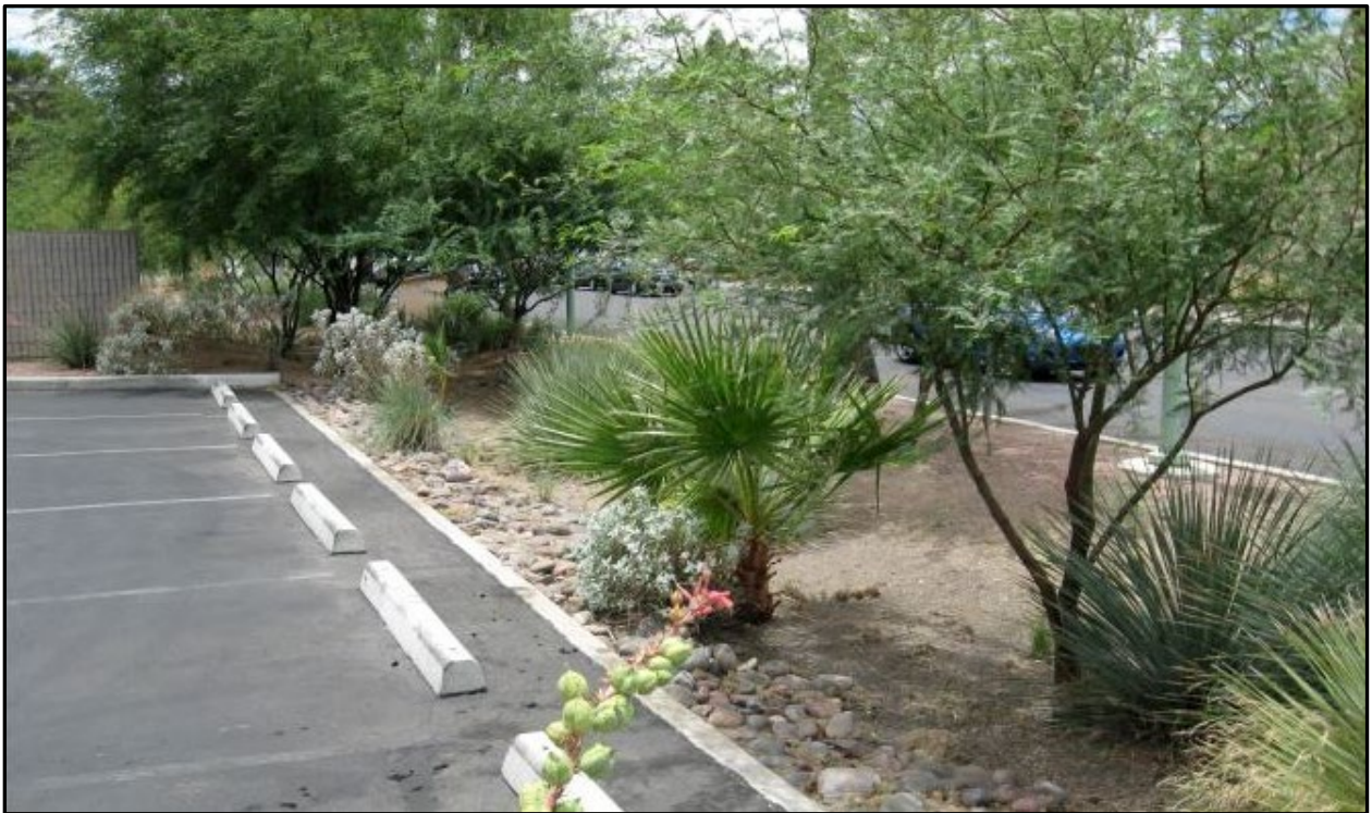
Figure 2-16. Flush Curb at Edge of Asphalt Parking Lot
