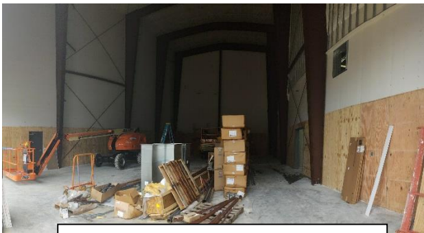
Apparatus Repair Bays
