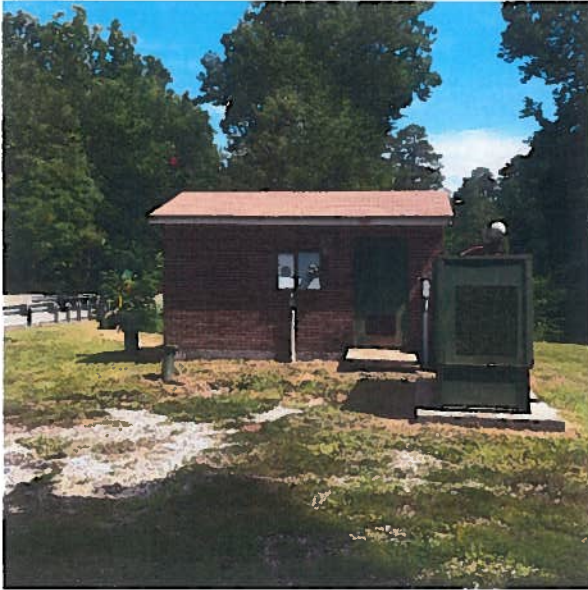
Image 1. Pump station exterior.
