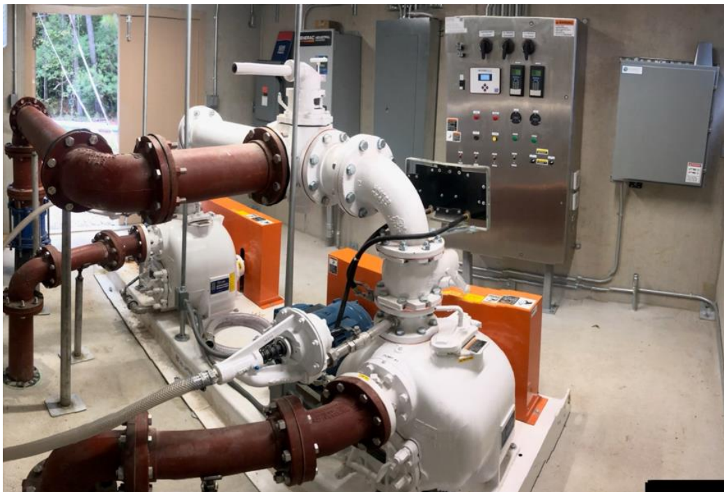
Richard Bland Pump Station (#7) – new pumps, pipes, SCADA and control panel- completed December 2021.
