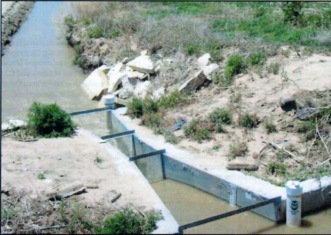
Figure 13. Permanent measurement structure for inflow to Field DS6, provided by Fort Lyon Canal Company during seasons 2005-2008
