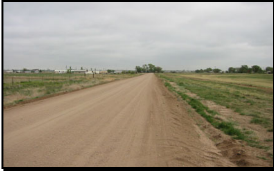
Typical unpaved County road with no shoulder.
