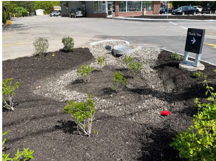
View of stormwater BMP installed at 524 Main Street
