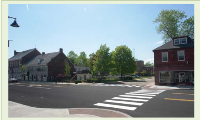
Main Street Renovations - new sidewalks, landscaping - street lights and paving.
