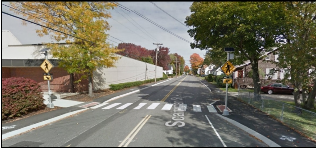
Scammon Street – Pedestrian Bumpout and Rectangular Rapid Flashing Beacon
