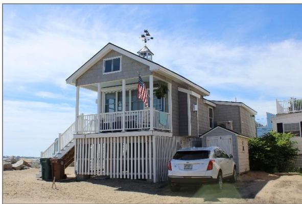
Example of raised structure at 7 Pearl Avenue
