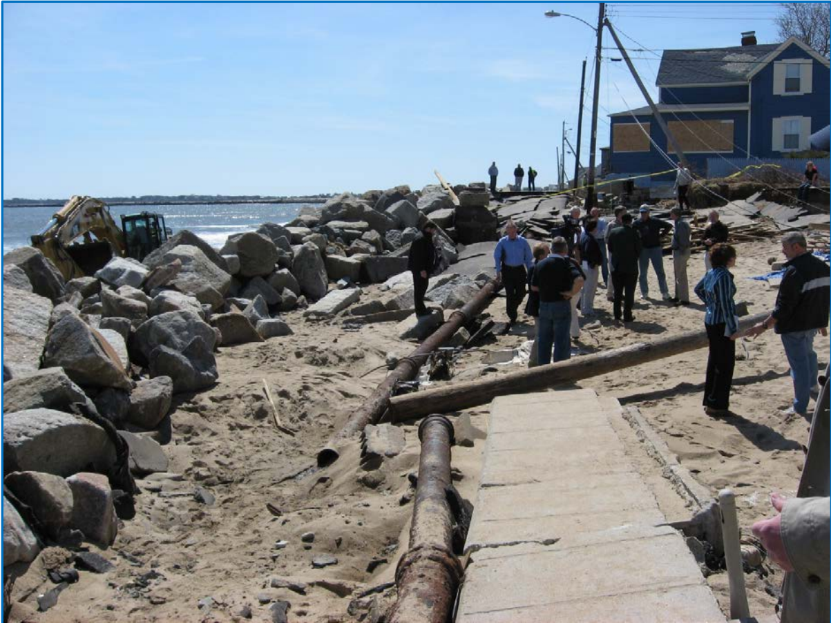
Figure 6 – Damage along Surf Street, Patriot’s Day storm of 2007
