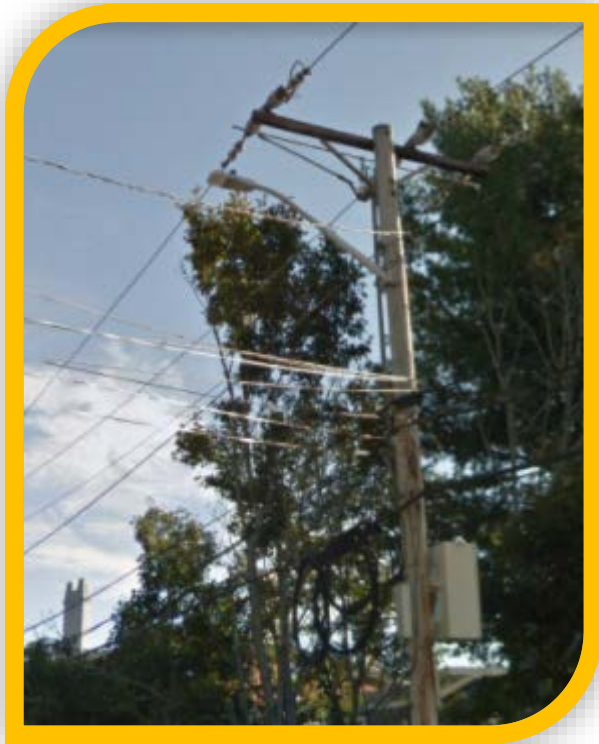
Our project in Newbury, MA
