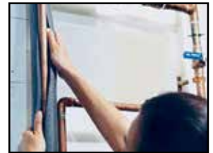
Pipe insulation, used to wrap any outside exposed pipes.
