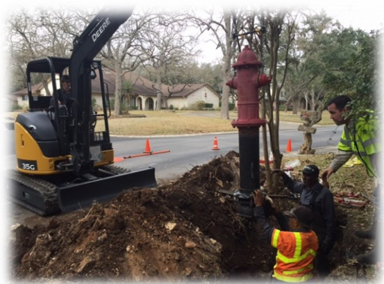
Public Works crew replacing a fire hydrant
