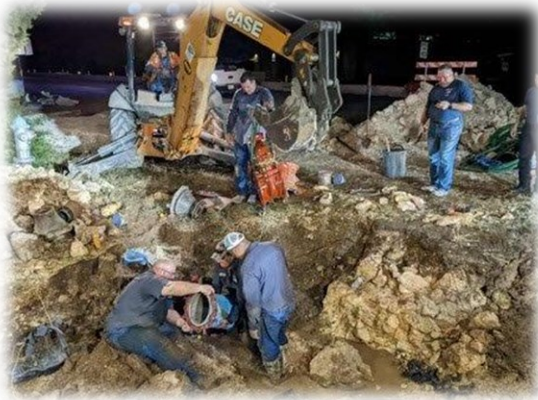
Public Works crew repairing a water main break on NW Military
