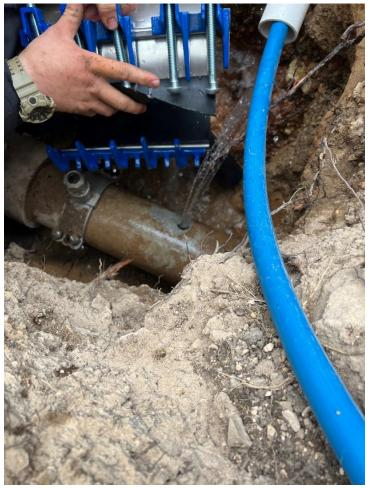
You can see the repair clamp in the top of the picture that is going around the pipe. This will seal off the flaked area for the service line to be installed without leaking. Cost difference between a saddle = \$56 and repair clamp with 1" tap = \$250
