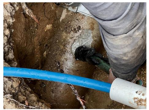
After taking the corporation out of the pipe, you can see if flaked the right side of the hole. A pipe was reinserted due to the hole filling up with water and we were getting a pump set up to suck the water out. Also the white pipe is the sleeve going under the roadway, with the new blue munipex pipe coming out to tie into the main.
