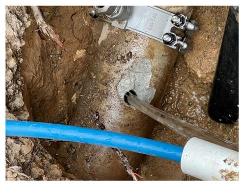
After cleaning the hole out we tried to install the new saddle that you can see in the top of the piture. The saddle is to small thus we needed to install a repair clamp with a 1" tap on it for the service hole to be reused.
