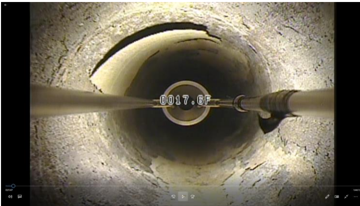
Casing at 17 ft with significant corrosion and delamination (or failed liner)
