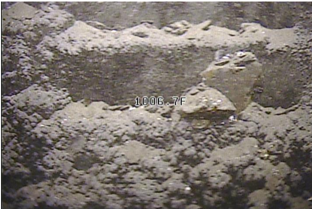
Casing slots at 1006 ft bgl bottom of screened interval with heavy precipitation
