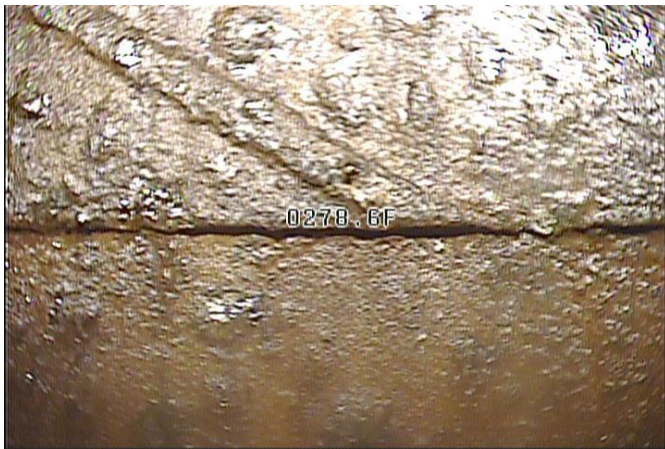
Casing at 278 ft bgl. View of helical-wound fabrication line and field welded pipe splice
