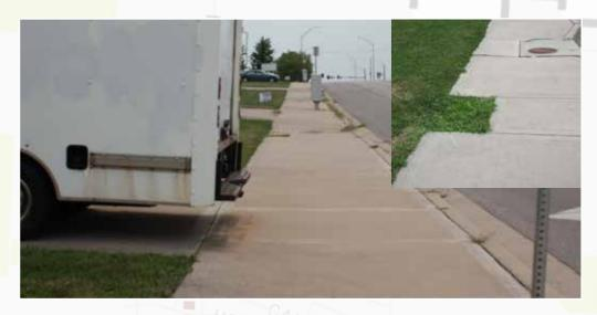
Wide sidewalk with a number of obstacles: sign posts, truck bumper, pavement cut-outs, inlet covers and mailboxes. Recommendation: Add curb stop for parking space, fill in missing concrete areas, consider moving mailboxes and sign posts where possible.
