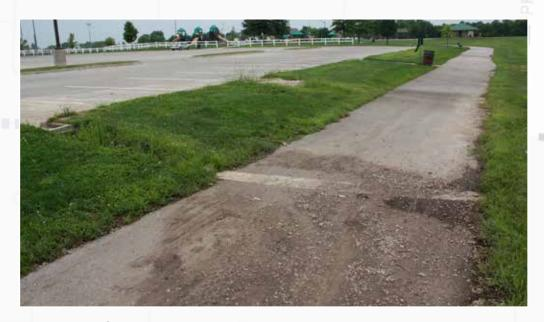
Stormwater from parking is overpowering drainage design. Maintenance has this location on their list to be addressed.
