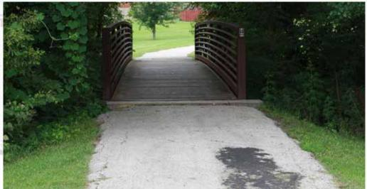
Good Parkway's asphalt is lifting over roots, cracking at culverts and sinking to make this elevation missmatch at a bridge abutment. Elevation adjustment already on Parks' winter project list. Recommendation: Replace Good Parkway asphalt trail segments with new cross-section standard.
