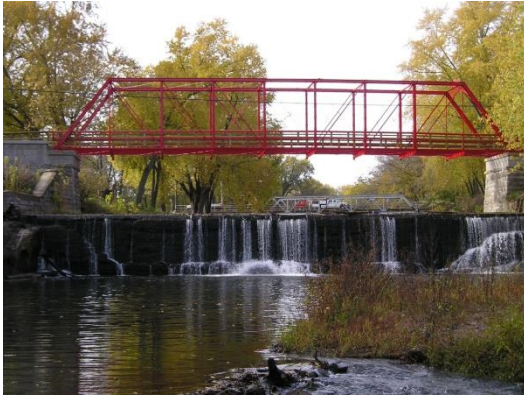
Restoration of the Old Appleton Bridge Village of Old Appleton
