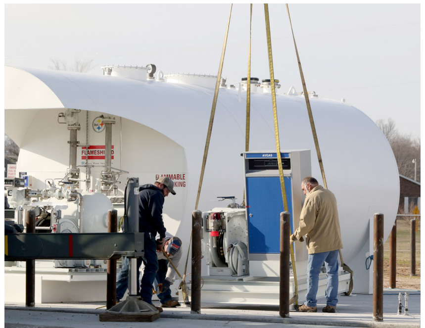
The project to install new fuel tanks was completed in 2023.
