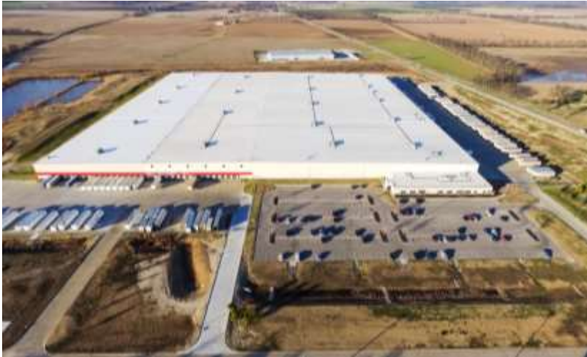
ORGILL DISTRIBUTION - $8 MILLION EXPANSION
