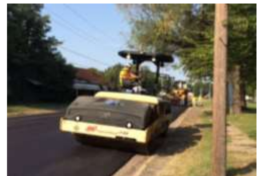
2015 ASPHALT STREET RESURFACING PROJECT
