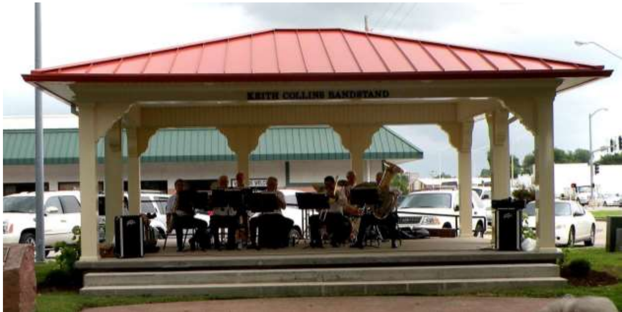
KEITH COLLINS BAND STAND, LEGION PARK, SIKESTON, CONSTRUCTED BY SIKESTON PUBLIC WORKS CREWS
