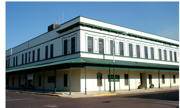
Sikeston City Hall, 105 E. Center Street
