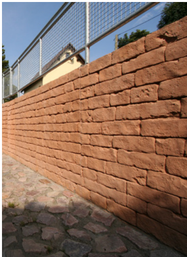
Brick formliner patterns could be used for the face of the culvert wing walls
