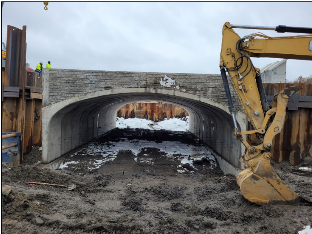
A milestone for the Davisburg Road/ Mill Pond Dam project was met in late January with the installation of this open bottom concrete culvert that will span the Shiawassee river.
