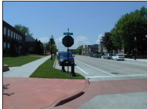
Curb extensions along Grant Street in De Pere
