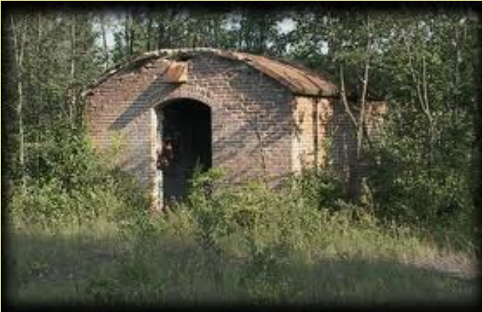
Example of Typical Brick Powder House
