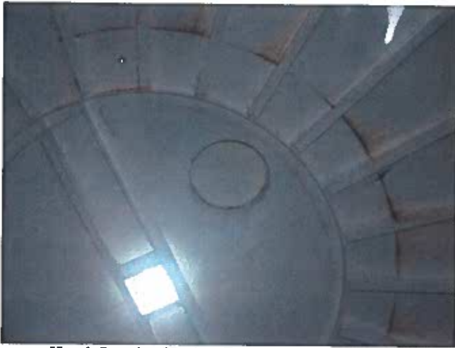
43 Hatch Interior Having Exposed Steel And Corrosion
