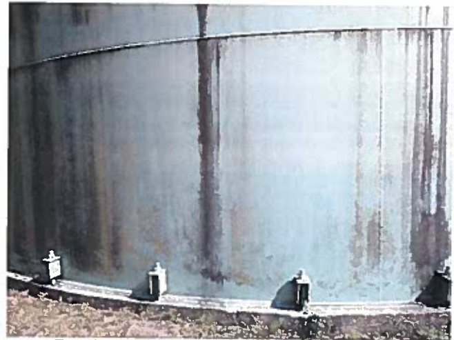
10 Exterior Wall Having Good Adhesion Value Of The Protective Coating And A Mild To Moderate Non-Uniform Accumulation Of Mildew
