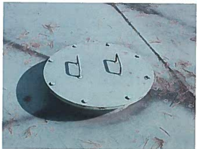
30 Hatch Secured With Nuts And Bolts
