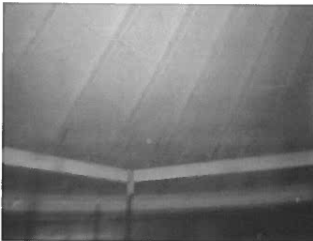
53 Overhead Panel Edges And Supports Having Corrosion Bleed-Through (Botch Rusting)
