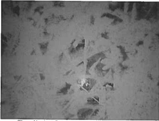
49 Floor Having Good Adhesion Value Of The Coating And A Mild To Moderate Stain
