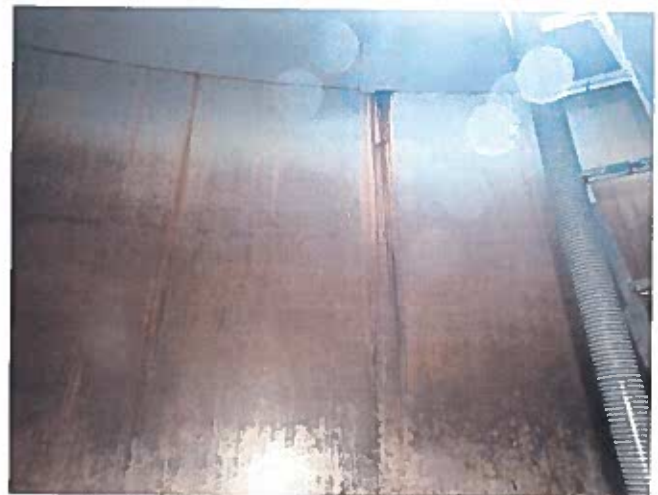
72 Top Of The Top Row Of Wall Panels At The Junction Of Where The Walls And Roof Meet Having Exposed Steel And Corrosion
