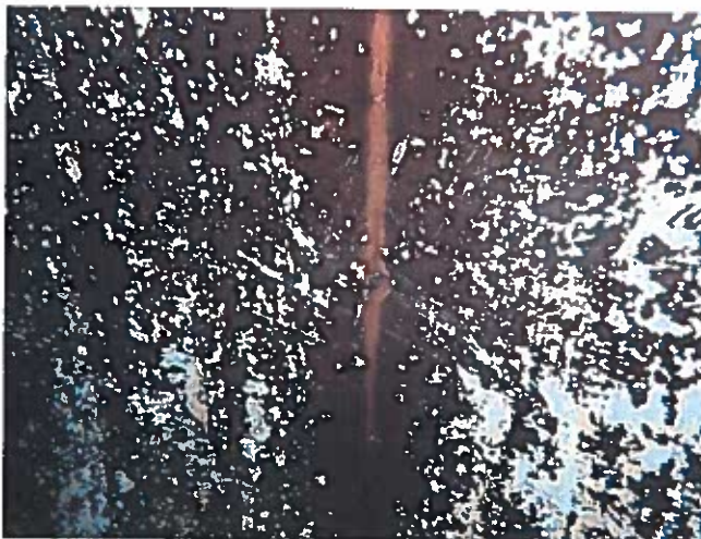
59 Interior Wall Having Coating Loss, Exposed Steel And Corrosion
