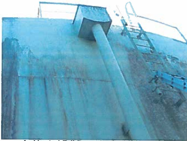
15 Ladder And Fall Prevention Device Having Good Adhesion Value Of The Coating
