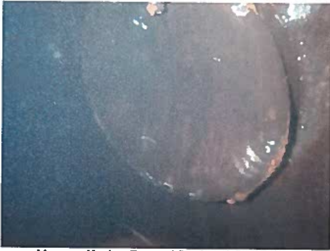
37 Manway Having Exposed Steel And Corrosion
