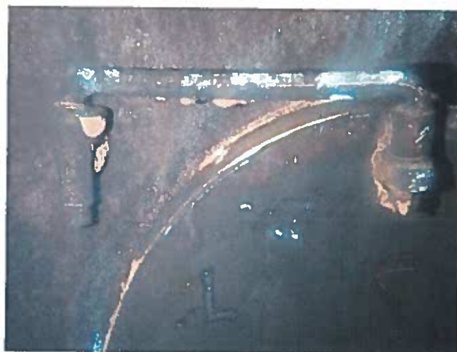
36 Manway Having Exposed Steel And Corrosion
