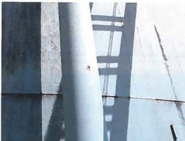
27 Overflow Pipe Having Exposed Steel And Corrosion
