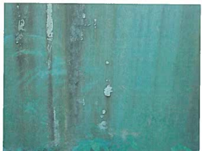
6 Exterior Wall Having Adhesion Loss Of The Finish Coating, Exposed Primary Coating And A Non-Uniform Accumulation Of Mildew
