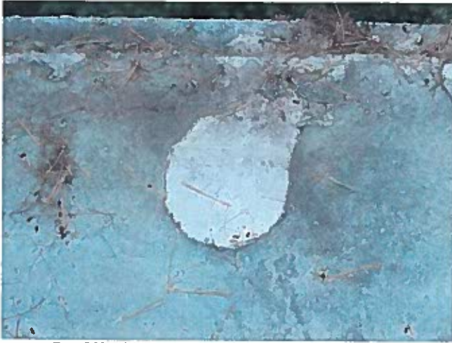
19 Roof Having Adhesion Loss Of The Finish Coat, Exposed Primary Coating, And A Non-Uniform Accumulation Of Mildew
