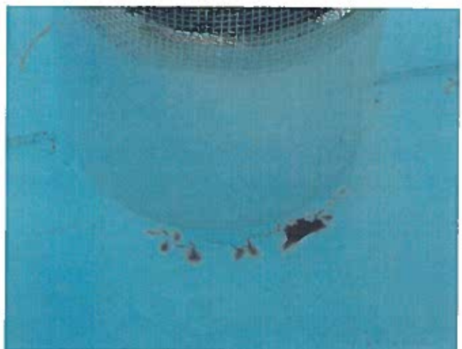
24 Coating Loss, Exposed Steel and Corrosion Throughout The Vent Base
