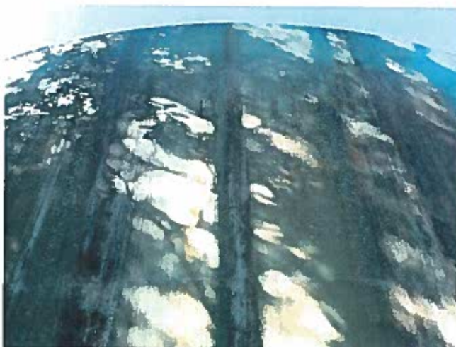
5 Exterior Wall Having Adhesion Loss Of The Finish Coating, Exposed Primary Coating And A Non-Uniform Accumulation Of Mildew
