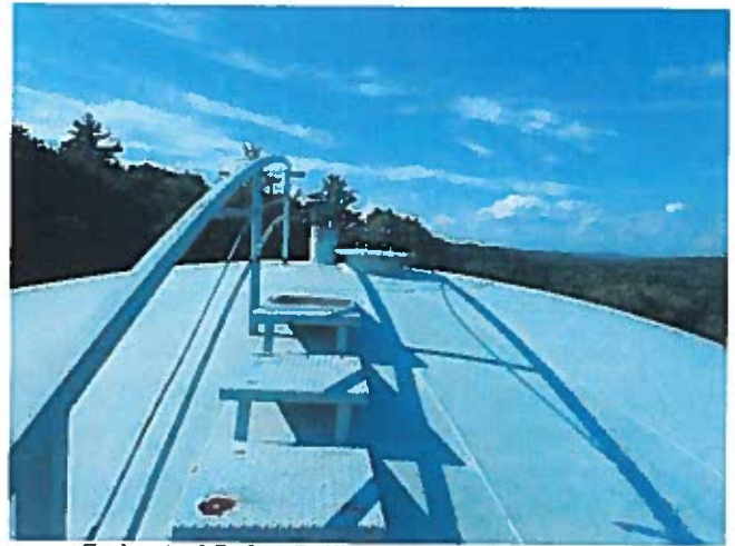
38 Stairs And Safety Railings Having Coating Loss, Exposed Steel And Corrosion
