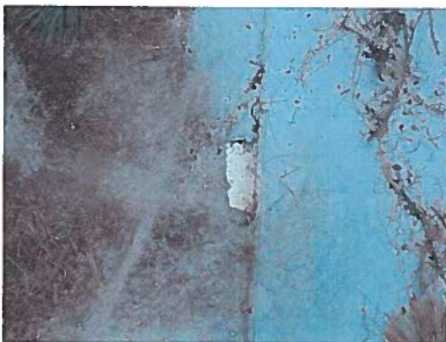
23 Roof Having Adhesion Loss Of The Finish Coat, Exposed Primary Coating, And A Non-Uniform Accumulation Of Mildew
