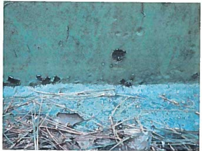
10 Exterior Wall Having Coating Loss, Exposed Steel, Corrosion And A Non-Uniform Accumulation Of Mildew
