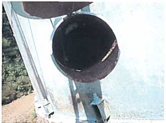
26 Unobstructed Overflow Pipe
