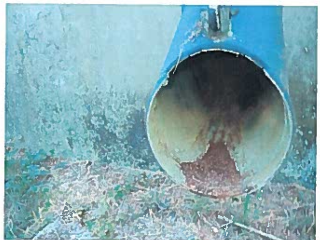
18 Overflow Pipe Found Unobstructed
