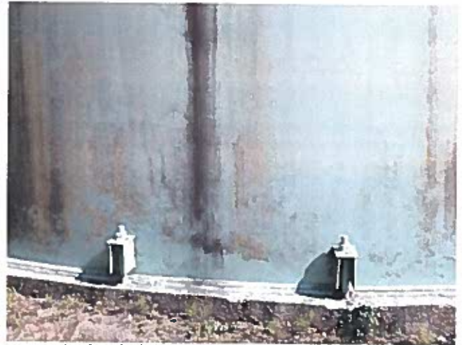
16 Anchor Bolt Assembly Having Exposed Steel And Corrosion
