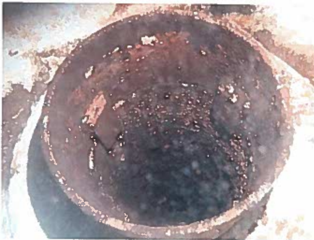
57 Removable Riser And Exposed Pipe Surfaces Having Exposed Steel And Corrosion
