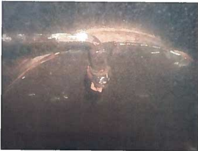
39 Manway Having Exposed Steel And Corrosion
