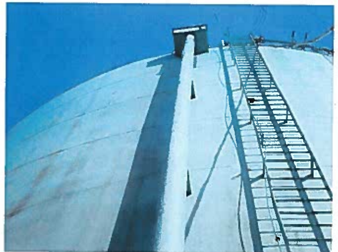
24 Overflow Weir Box And Overflow Pipe
