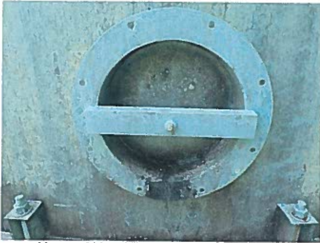
19 Manway Lid And Trunk Having Good Adhesion Value Of The Coating
