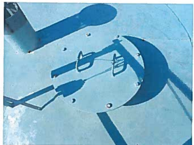
42 Hatch Exterior Having Exposed Steel And Corrosion
