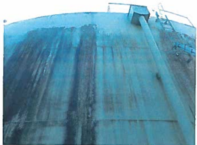
16 Overflow Weir Box And Overflow Pipe Having Good Adhesion Value Of The Coating
