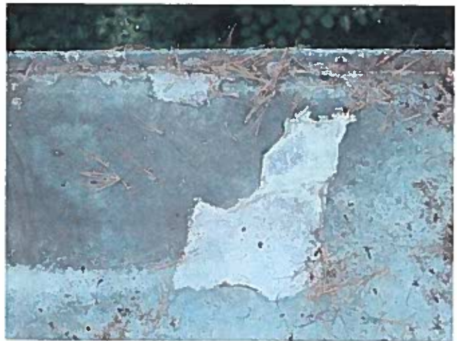
20 Roof Having Adhesion Loss Of The Finish Coat, Exposed Primary Coating, And A Non-Uniform Accumulation Of Mildew
