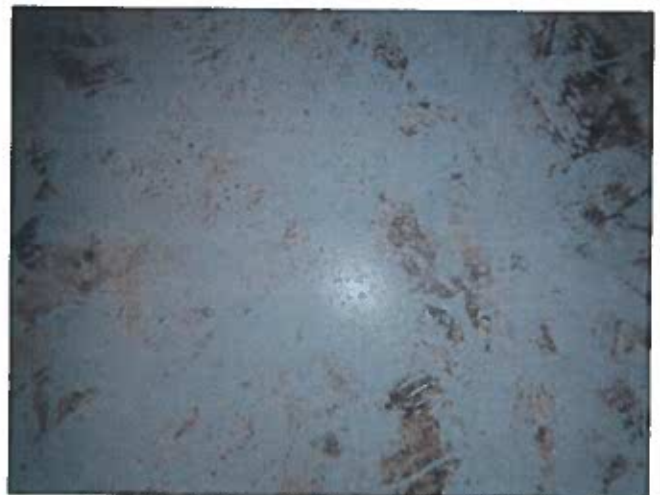
48 Floor Having Good Adhesion Value Of The Coating And A Mild To Moderate Stain
