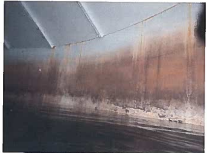
70 Top Of The Top Row Of Wall Panels At The Junction Of Where The Walls And Roof Meet Having Exposed Steel And Corrosion
