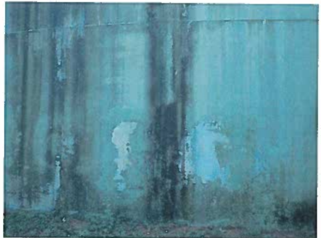
2 Exterior Wall Having Adhesion Loss Of The Finish Coating, Exposed Primary Coating And A Non-Uniform Accumulation Of Mildew
