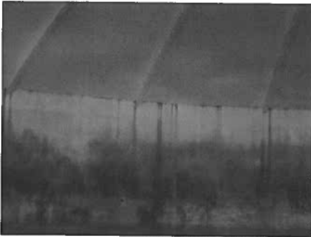
73 Top Of The Top Row Of Wall Panels At The Junction Of Where The Walls And Roof Meet Having Exposed Steel And Corrosion
