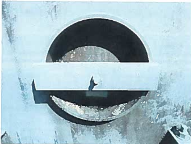
21 Manway Lid And Trunk Having Good Adhesion Value Of The Coating
