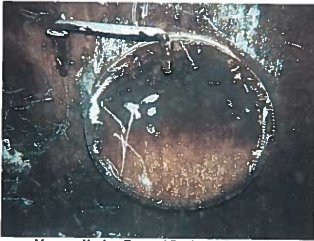
55 Manway Having Exposed Steel And Corrosion
