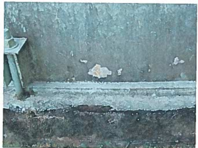
6 Exterior Wall Having Exposed Primary Coating
