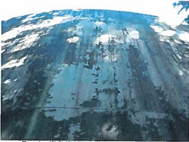
1 Exterior Wall Having Adhesion Loss Of The Finish Coating, Exposed Primary Coating And A Non-Uniform Accumulation Of Mildew
