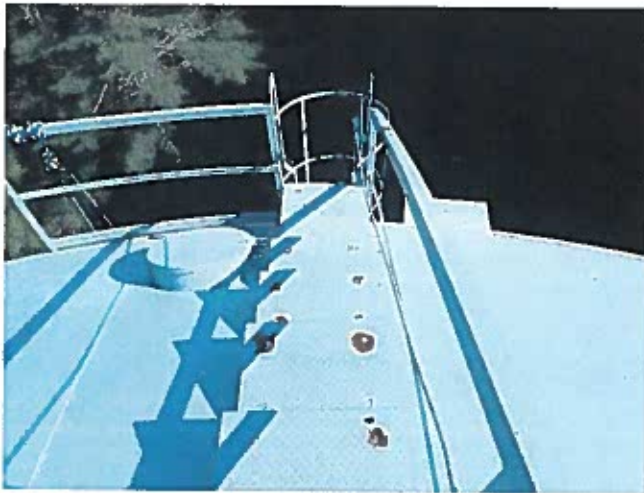
39 Stairs And Safety Railings Having Coating Loss, Exposed Steel And Corrosion
