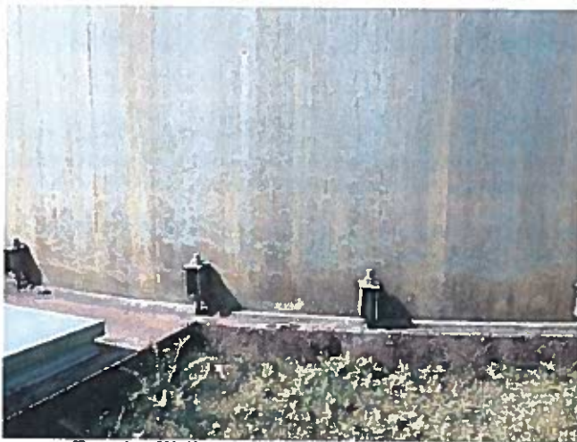
3 Exterior Wall Having Exposed Steel And Corrosion
