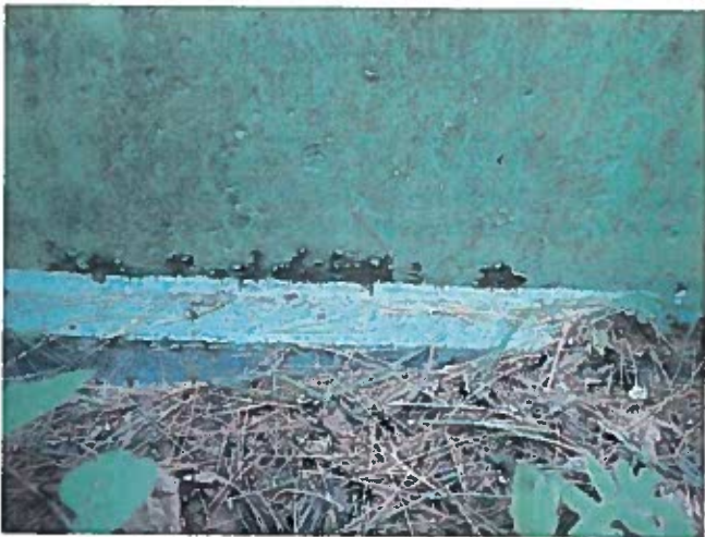
9 Exterior Wall Having Coating Loss, Exposed Steel, Corrosion And A Non-Uniform Accumulation Of Mildew
