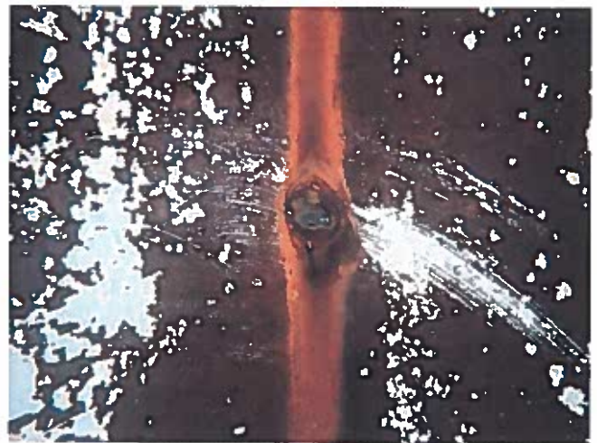
62 Interior Wall Having Coating Loss, Exposed Steel And Corrosion
