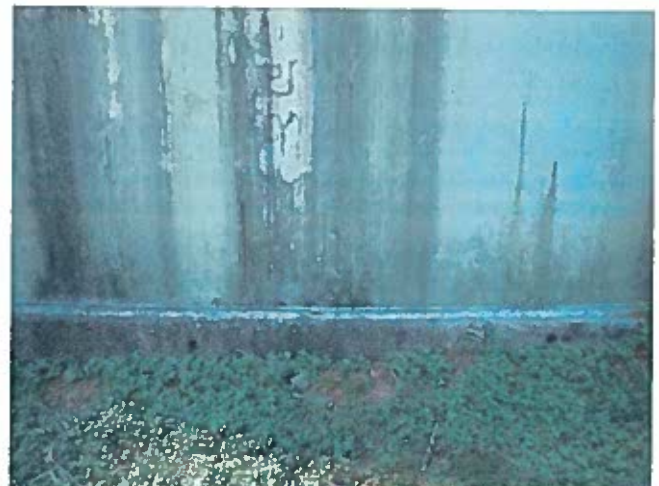
4 Exterior Wall Having Adhesion Loss Of The Finish Coating, Exposed Primary Coating And A Non-Uniform Accumulation Of Mildew
