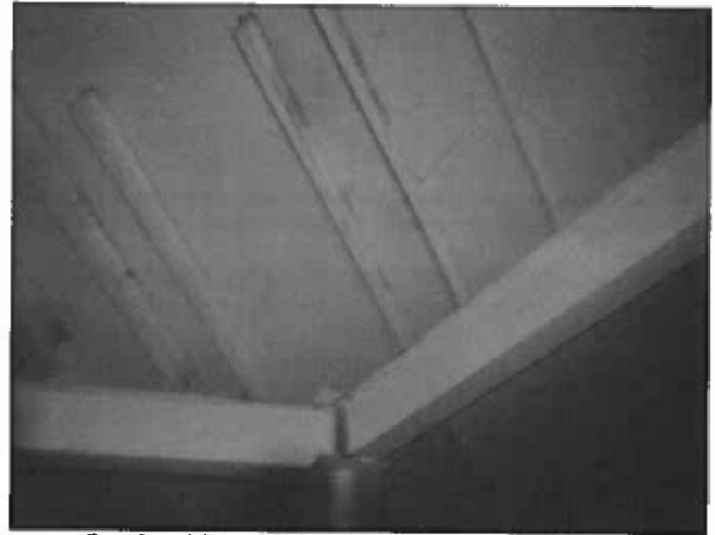
52 Overhead Panel Edges And Supports Having Corrosion Bleed-Through (Botch Rusting)
