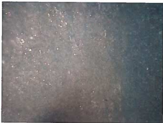
43 Interior Wall Having A Heavy Stain To A Film Of Precipitate
