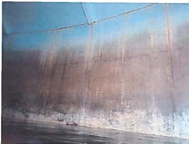
71 Top Of The Top Row Of Wall Panels At The Junction Of Where The Walls And Roof Meet Having Exposed Steel And Corrosion
