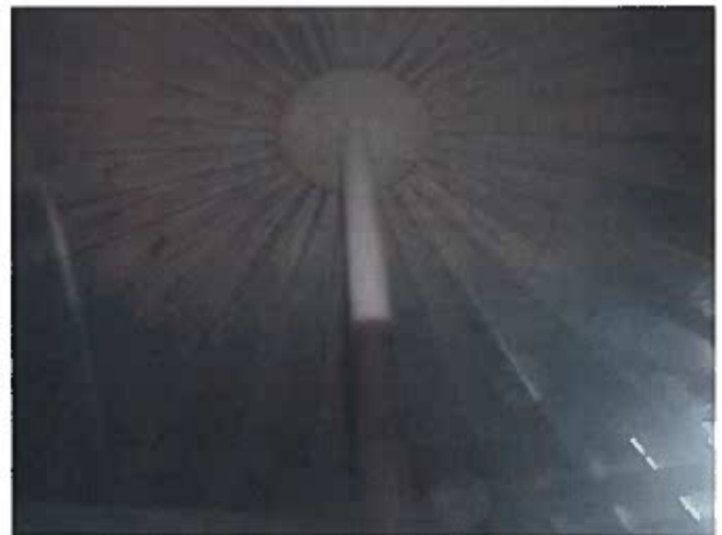
64 Support Column Having Good Adhesion Value Of The Coating And A Heavy Stain To A Film Of Precipitate
