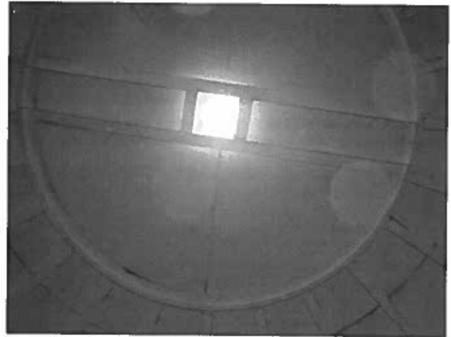
76 Overhead Panels, Welds And Supports Having Corrosion Bleed-Through
