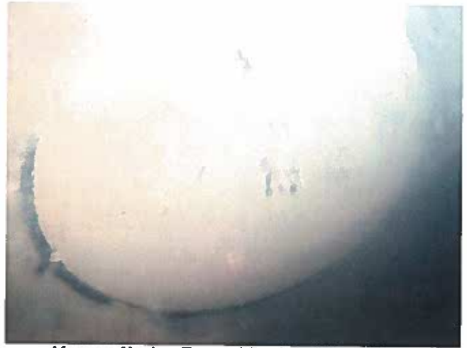
38 Manway Having Exposed Steel And Corrosion
