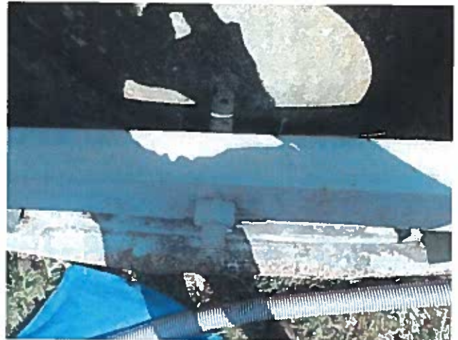
22 Manway Securing Nut And Bolt Having Corrosion
