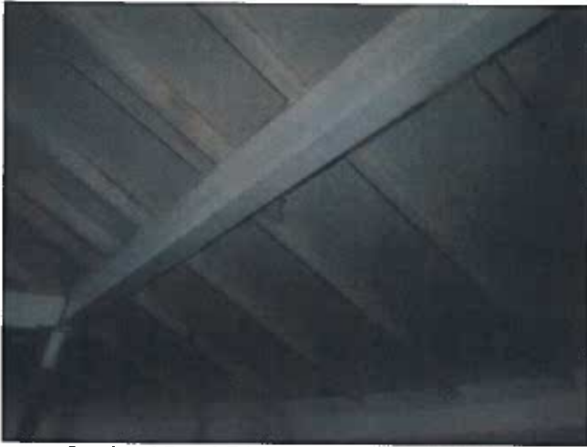
55 Overhead Panel Edges And Supports Having Corrosion Bleed-Through (Botch Rusting)
