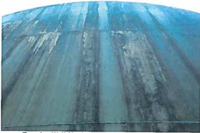
7 Exterior Wall Having Adhesion Loss Of The Finish Coating, Exposed Primary Coating And A Non-Uniform Accumulation Of Mildew
