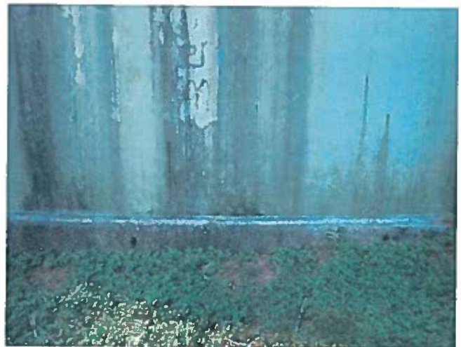
12 Exposed Foundation Surfaces Appearing Sound
