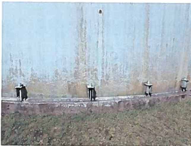
17 Anchor Bolts Having Good Adhesion Value Of The Protective Coating
