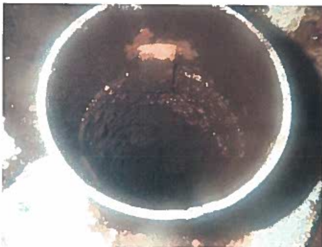
41 Interior Surfaces Of The Pipe Having Exposed Steel And Corrosion
