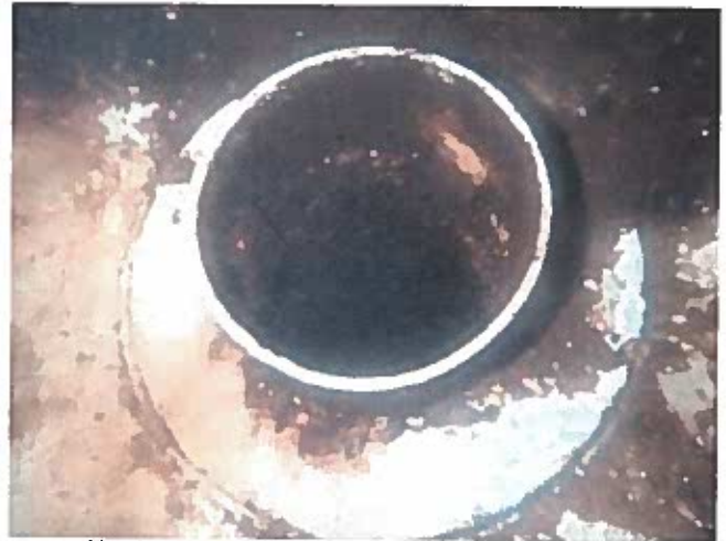
40 Unobstructed Influent/Effluent Pipe
