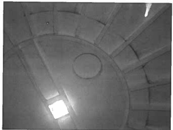
78 Overhead Panels, Welds And Supports Having Corrosion Bleed-Through
