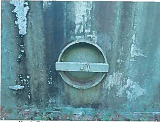
13 North-Easternmost Manway Having Minimal Steel Exposure On The Securing Hardware
