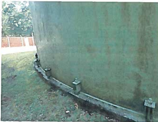
9 Exterior Wall Having Good Adhesion Value Of The Protective Coating And A Mild To Moderate Non-Uniform Accumulation Of Mildew
