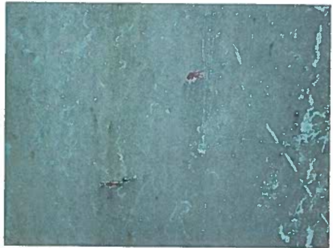
8 Exterior Wall Having Coating Loss, Exposed Steel, Corrosion And A Non-Uniform Accumulation Of Mildew
