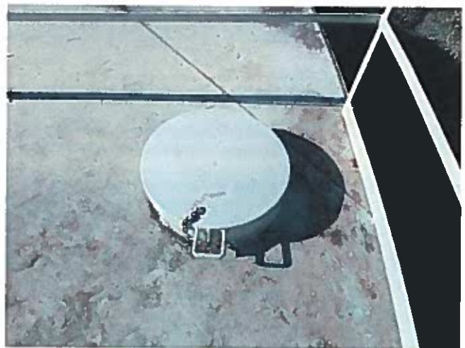
28 Hatch Exterior Having Exposed Steel And Corrosion
