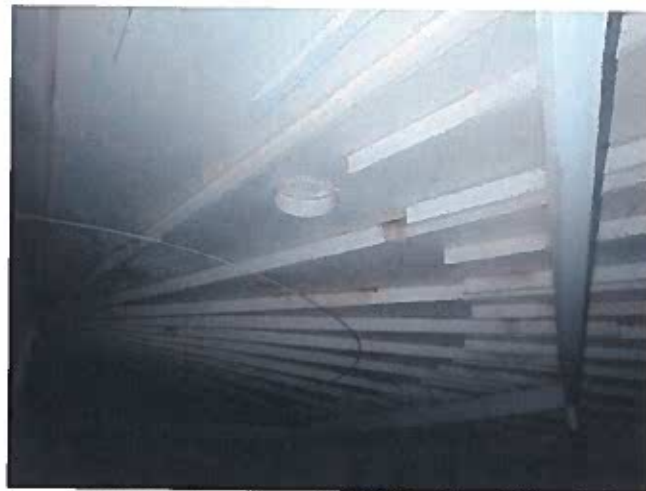
32 Hatch Interior Appearing To Have Good Adhesion Value Of The Protective Coating
