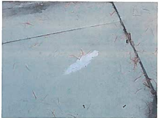
22 Roof Having Adhesion Loss Of The Finish Coat, Exposed Primary Coating, And A Non-Uniform Accumulation Of Mildew
