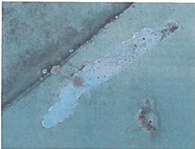
21 Roof Having Adhesion Loss Of The Finish Coat, Exposed Primary Coating, And A Non-Uniform Accumulation Of Mildew
