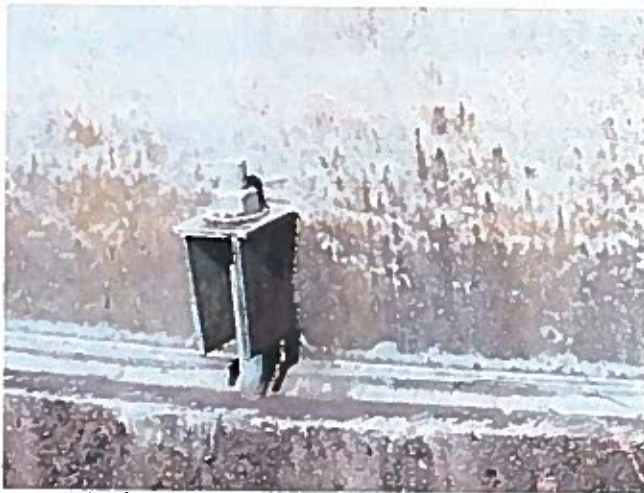
15 Anchor Bolt Assembly Having Exposed Steel And Corrosion
