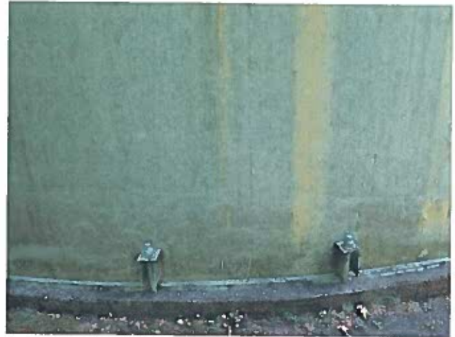
8 Exterior Wall Having Good Adhesion Value Of The Protective Coating And A Mild To Moderate Non-Uniform Accumulation Of Mildew
