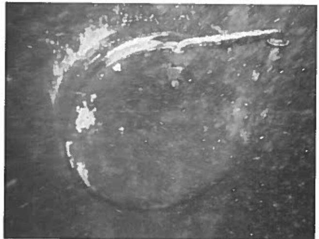
54 Manway Having Exposed Steel And Corrosion
