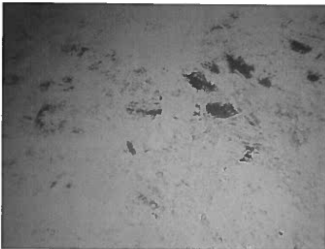
53 Floor Having Good Adhesion Value Of The Coating And A Mild To Moderate Stain
