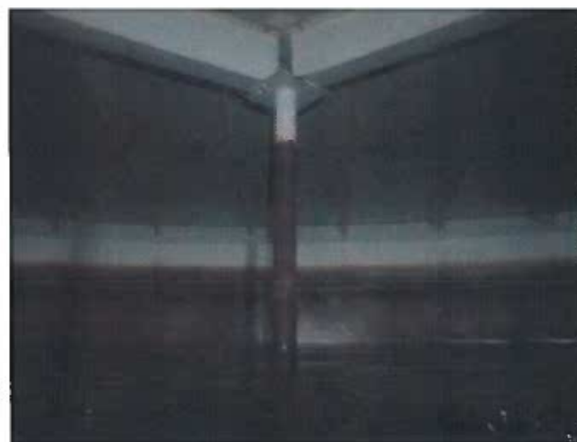
65 Support Column Having Good Adhesion Value Of The Coating And A Heavy Stain To A Film Of Precipitate
