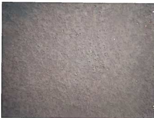
44 Interior Wall Having A Heavy Stain To A Film Of Precipitate
