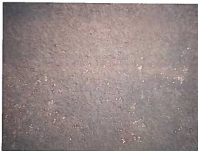
46 Interior Wall Having A Heavy Stain To A Film Of Precipitate
