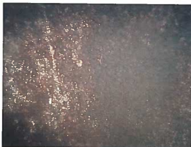
48 Interior Wall Having A Heavy Stain To A Film Of Precipitate
