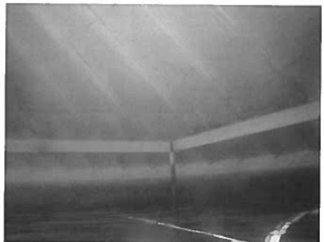
54 Overhead Panel Edges And Supports Having Corrosion Bleed-Through (Botch Rusting)
