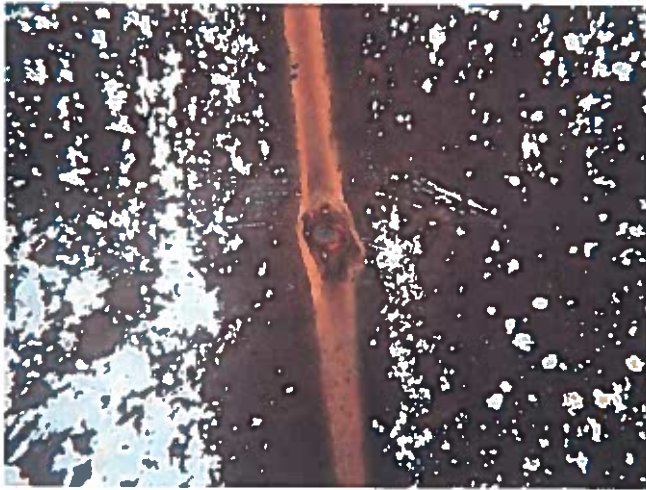
61 Interior Wall Having Coating Loss, Exposed Steel And Corrosion
