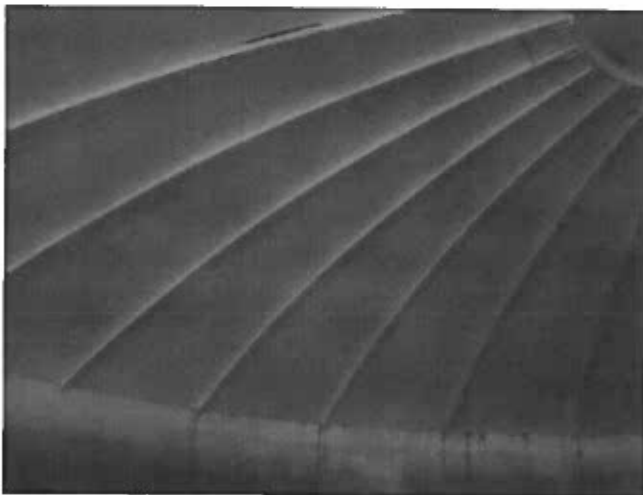
77 Overhead Panels, Welds And Supports Having Corrosion Bleed-Through
