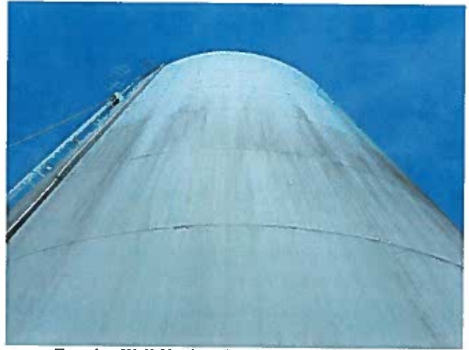
14 Exterior Wall Having Good Adhesion Value Of The Protective Coating And A Mild To Moderate Non-Uniform Accumulation Of Mildew
