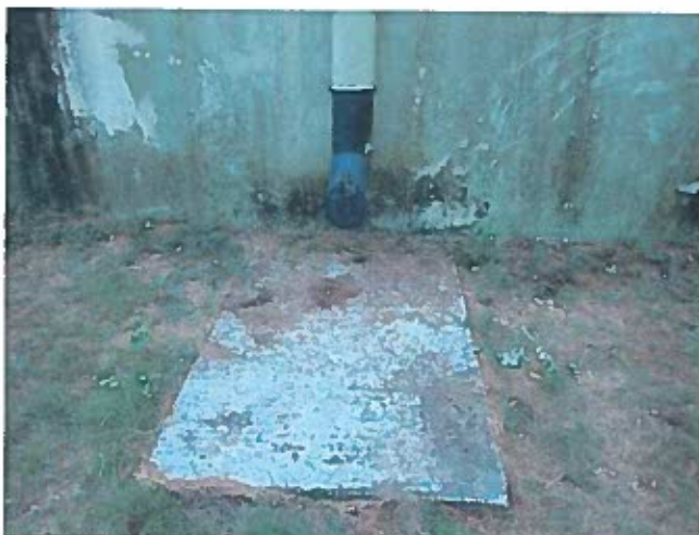
17 Overflow Pipe Terminating Above A Concrete Splash Pad
