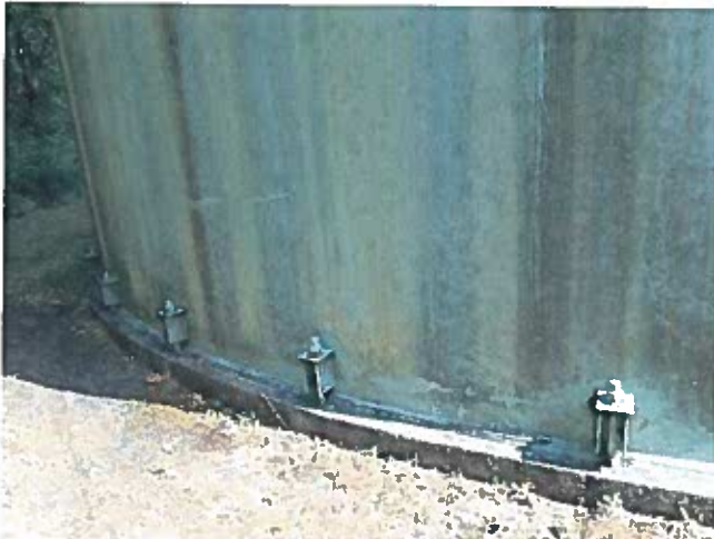
7 Exterior Wall Having Good Adhesion Value Of The Protective Coating And A Mild To Moderate Non-Uniform Accumulation Of Mildew
