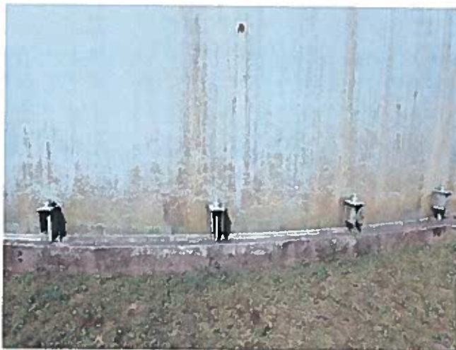
5 Exterior Wall Having Exposed Steel And Corrosion
