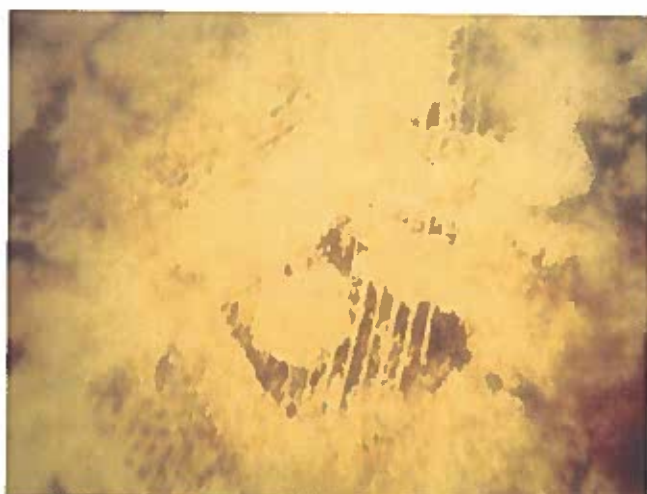
35 Floor Having Good Adhesion Value Of The Protective Coating And A Mild To Moderate Stain
