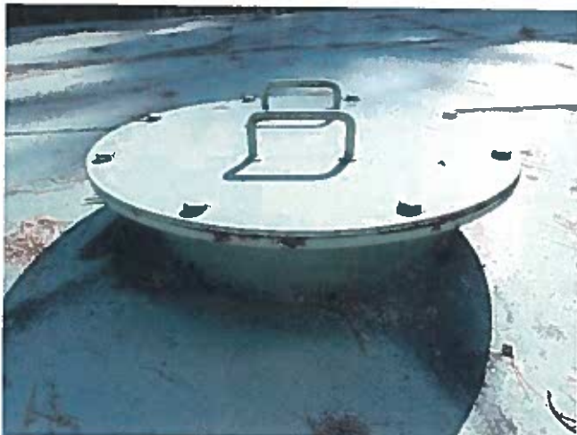
31 Hatch Exterior Having Exposed Steel And Corrosion
