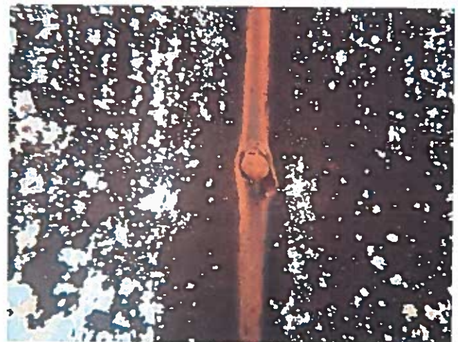
60 Interior Wall Having Coating Loss, Exposed Steel And Corrosion
