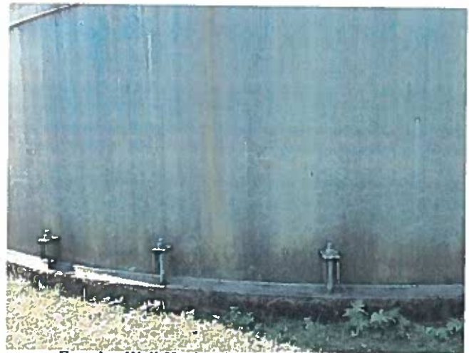
4 Exterior Wall Having Exposed Steel And Corrosion
