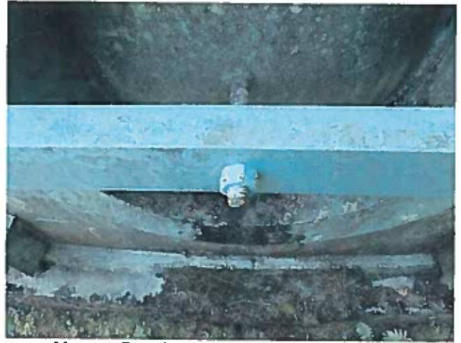
20 Manway Securing Nut And Bolt Having Corrosion
