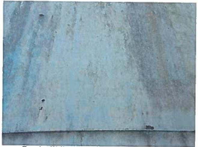
2 Exterior Wall Having Exposed Steel And Corrosion
