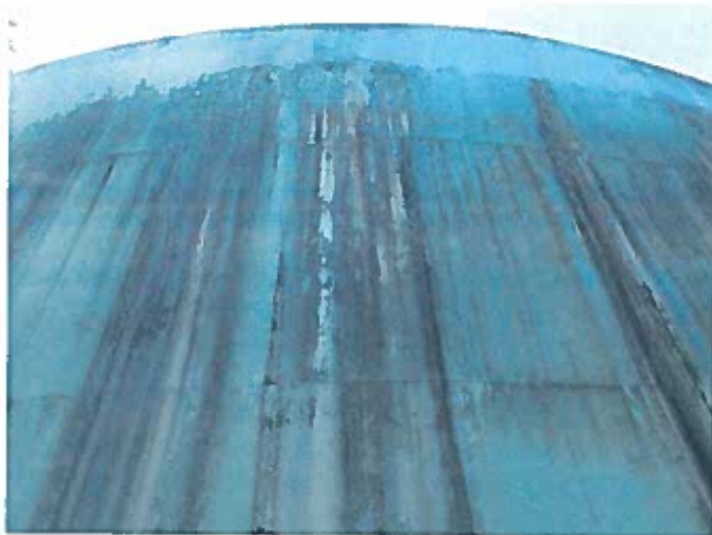
3 Exterior Wall Having Adhesion Loss Of The Finish Coating, Exposed Primary Coating And A Non-Uniform Accumulation Of Mildew
