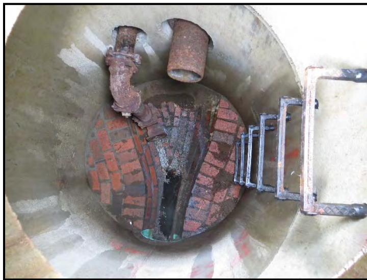
FIGURE 2-6 GIBBS CROSSING PUMPING STATION DISCHARGE MANHOLE
