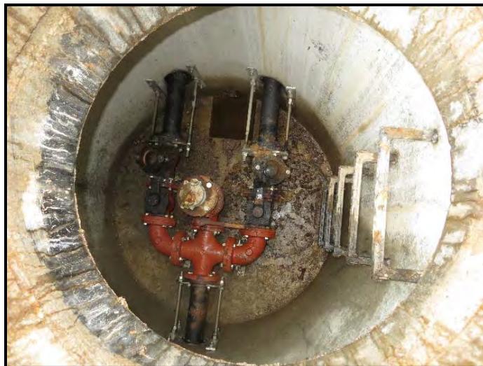
FIGURE 2-5 GIBBS CROSSING PUMPING STATION VALVE PIT AND BYPASS CONNECTION
