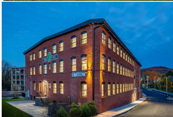
3 Ferry Street, Easthampton, from MassLive (during demolition) and 3 Ferry Street - One Ferry Project
