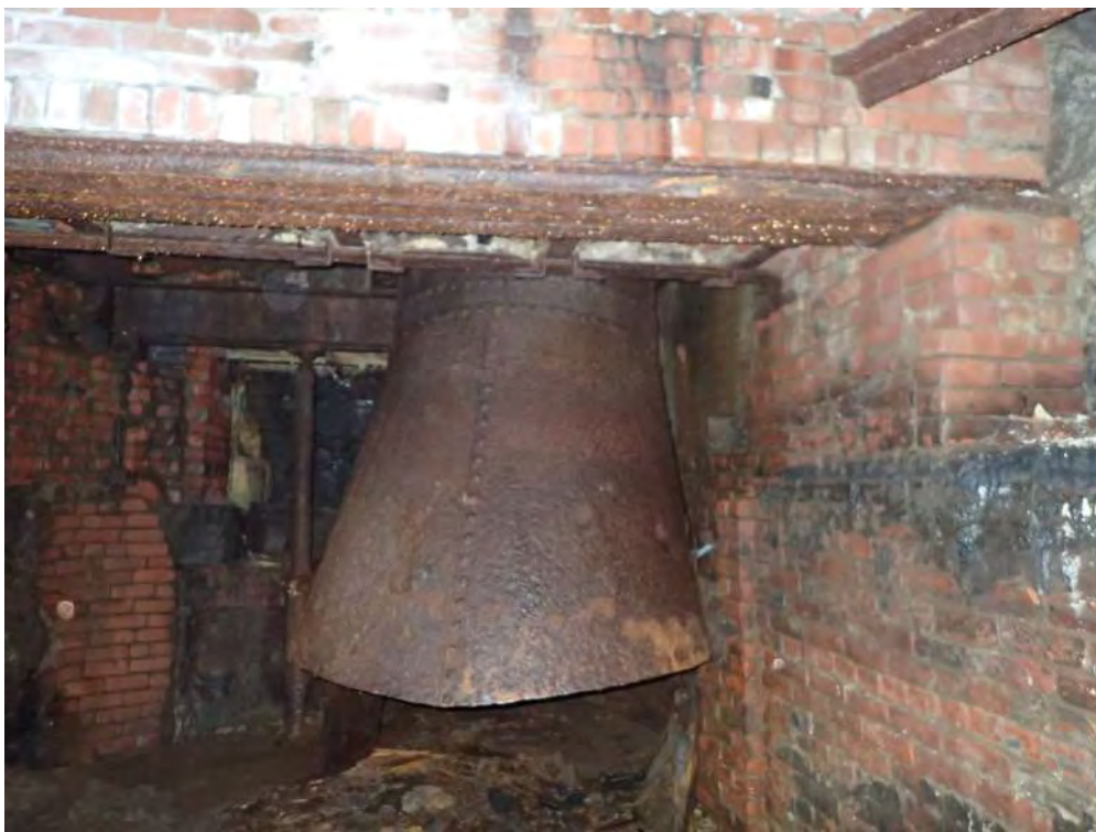
Photo 10: Alcove in Northern Portion of Tunnel with Steel Drain
