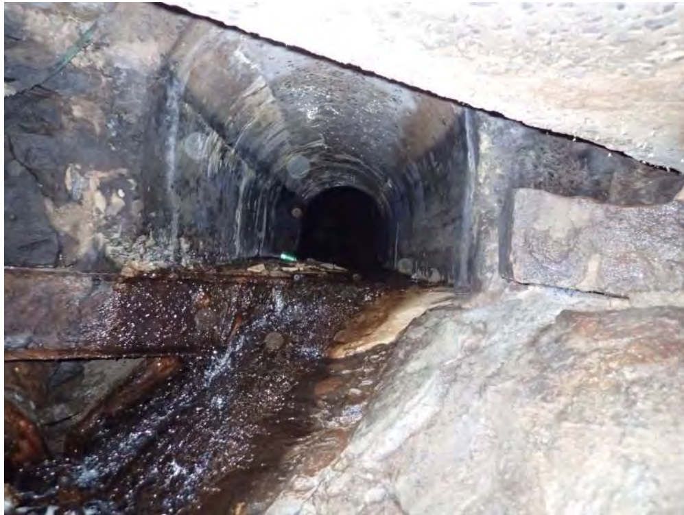
Photo 05: Formed Concrete Tunnel – North Side of Main Tunnel – Active Water Flow
