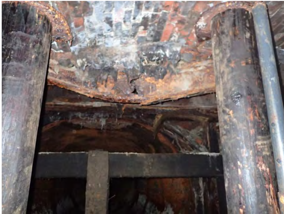
Photo 01: Supplemental Support at West End Culvert Intersection
