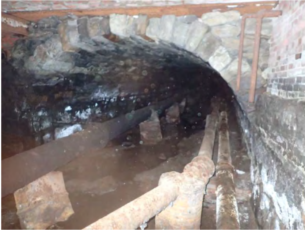
Photo 11: Granite Arch Portion of Tunnel
