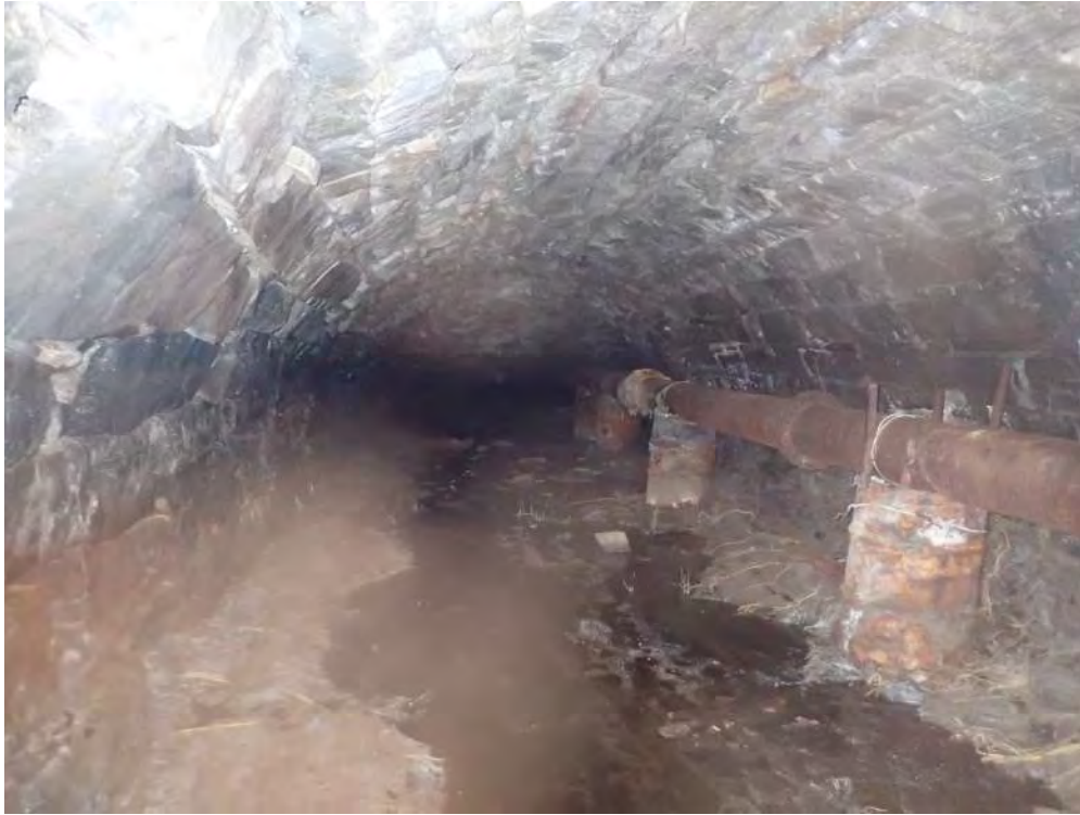
Photo 13: Second East – West Tunnel Portion – Stone Arch Construction
