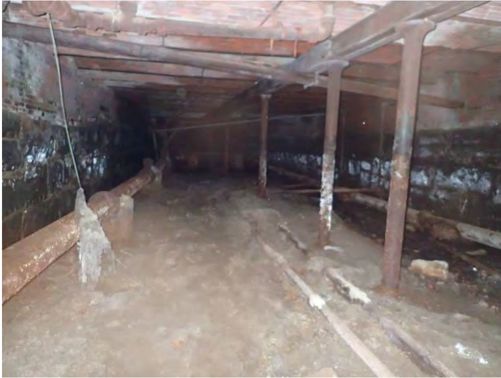
Photo 09: Center Line of Support Columns Along Northerly Portion of Tunnel
