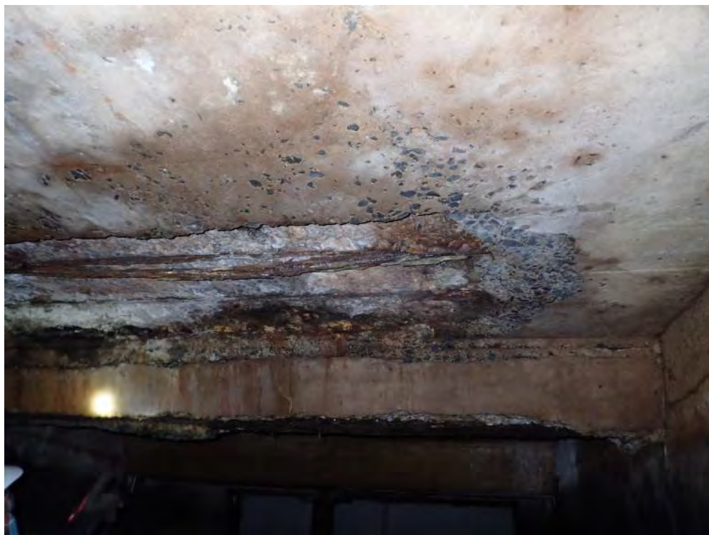
Photo 04: Exposed Concrete Reinforcing with Steel Beam Showing Section Loss
