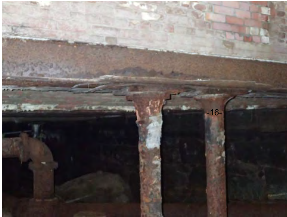
Photo 07: Support Beam and Columns at Tunnel Turn to the North
