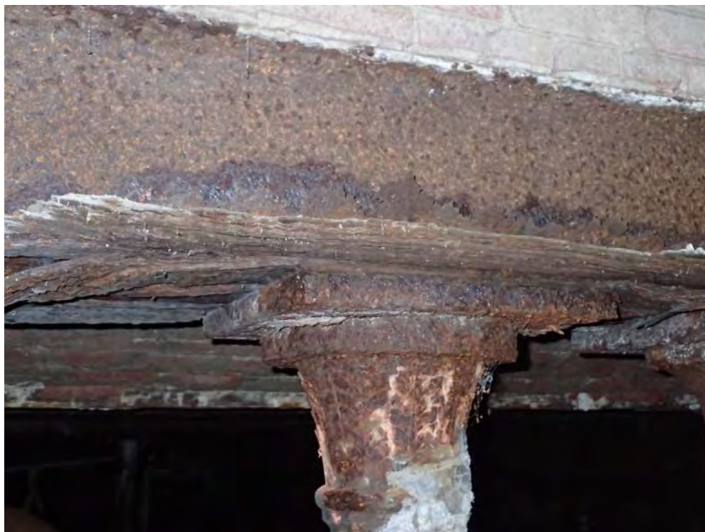
Photo 08: Support Column Deterioration at Tunnel Turn to the North
