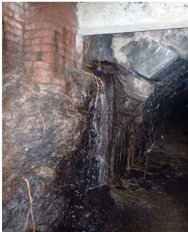
Photo 14: Transition from Stone Arch to Brick Masonry Construction – with Active Water Flow
