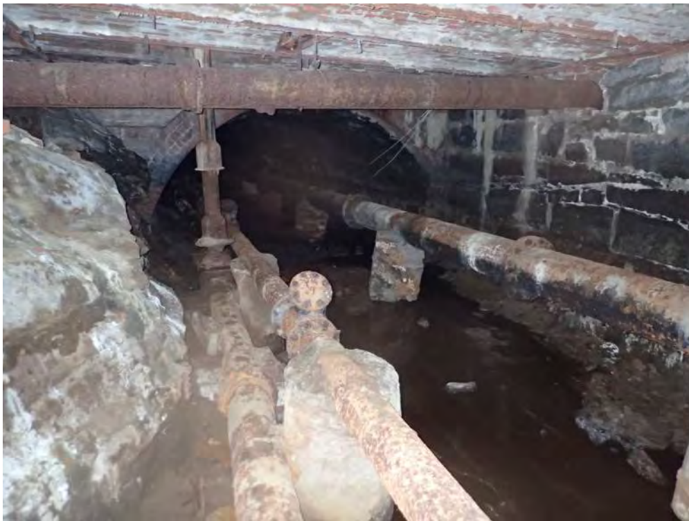
Photo 12: Bedrock Sidewall with Pipes Continuing Through Tunnel
