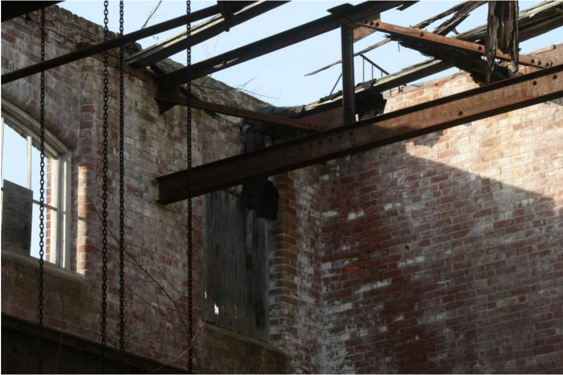
Photo 3: Upper Portion of Masonry Walls and Steel Roof Members
