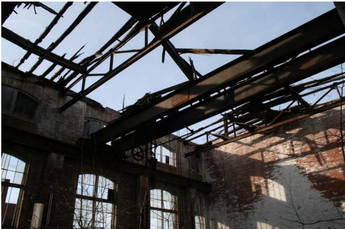
Photo 2: Failed Roof Deck of Building #9
