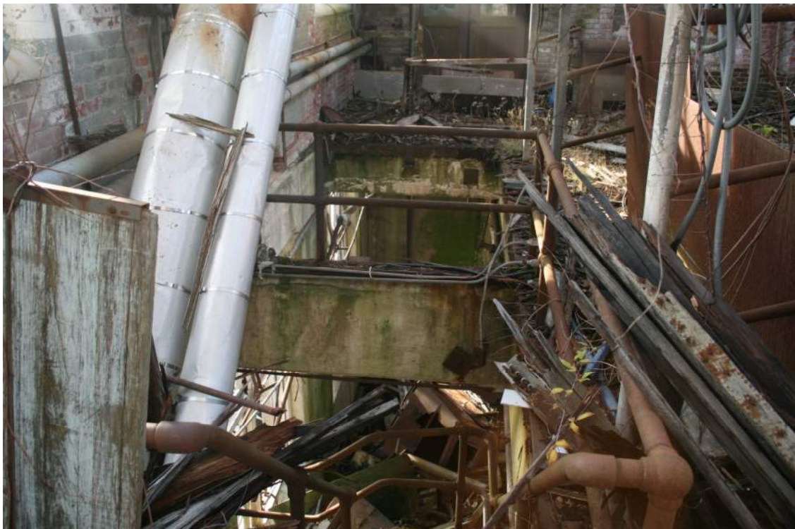
Photo 6: Evidence of Cast-in-Place Concrete Floor System
