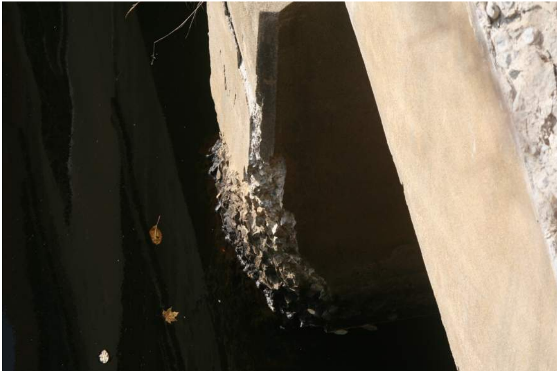
Photo 7: Deteriorated and Spalled Concrete Pilaster
