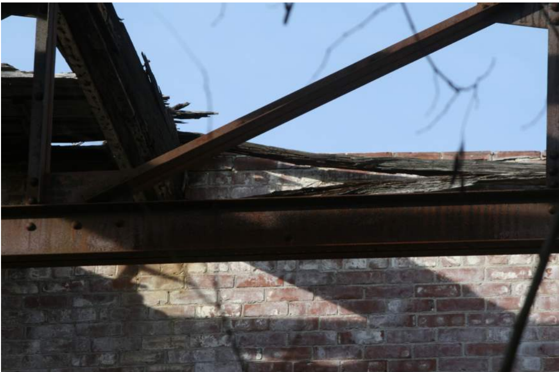
Photo 4: Surface Rust on Steel Roof Members
