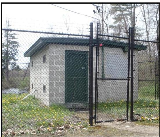
Well No. 4, which is also called the “Giard Well”, was constructed in 1965. Well No. 4 is an 18-inch by 24-inch gravel packed well that has a depth of approximately 51 feet and a well screen of 10 feet. The well is equipped with a vertical turbine pump that is powered by a 10 HP motor. The well is located approximately 800 feet southwest of Snow Pond off Pleasant Street, and the well is enclosed within a block well house that is protected with a black fence with barbed wire for security.
