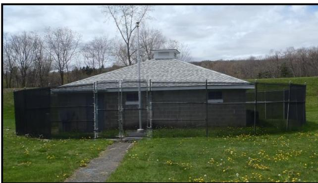
security with the use of a security camera is intended to be installed in the future. The floor of the well is a natural bottom that consists of stone and sand. The Cistern is currently permitted for a maximum authorized withdrawal of 330 gpm (0.475 MGD). The Cistern holds approximately 230,000 gallons when full.
