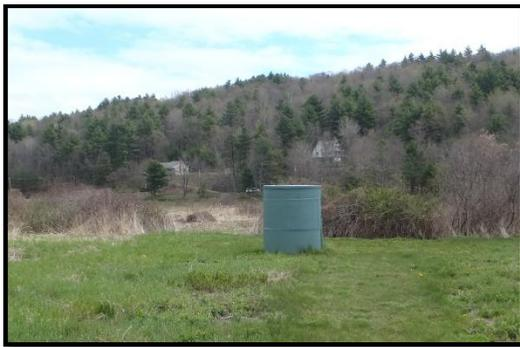
approximately 1,000 feet northwest of Gilbertville Road (Route 32). The well is a 12-inch by 18-inch gravel packed well that has a depth of approximately 68 feet and a well screen of 13 feet. The Dismal Swamp Well is protected by a concrete structure that is built around the casing since the well is located within the 100 year flood plain (as
