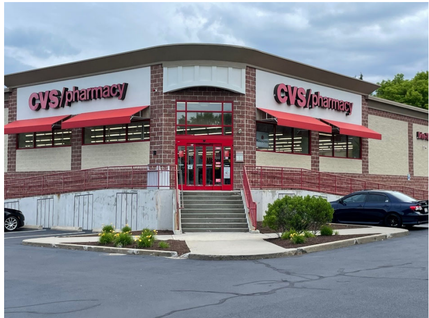
Figure 10. Elevated Construction. The entrance to the CVS on West Street illustrates elevated construction to minimize flooding risks. In addition to the stairwell, there are handicap access ramps on each side of the building to reach the store entrance.
