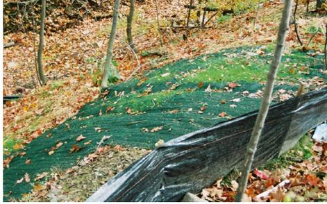
Figure 1: Turf Reinforcement Matting
