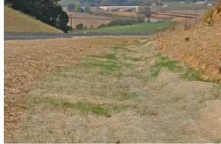
Figure 2: Erosion Control Matting
